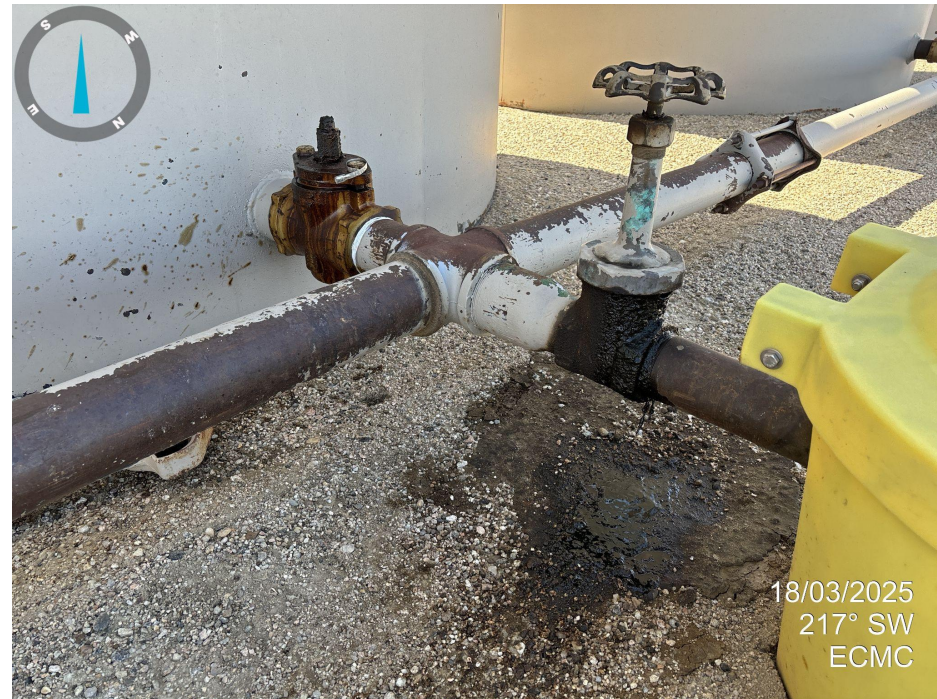
Photo 2. Valve is leaking. Stained soil is present beneath valve.
