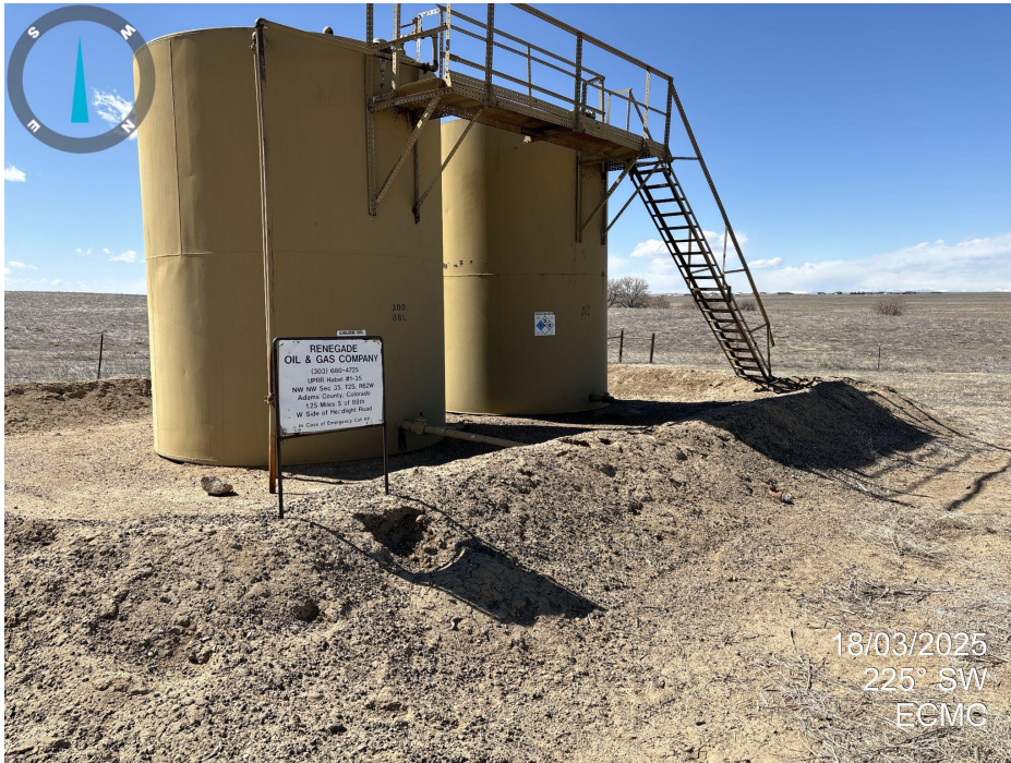
Photo 3. Tank battery looking southwest.
