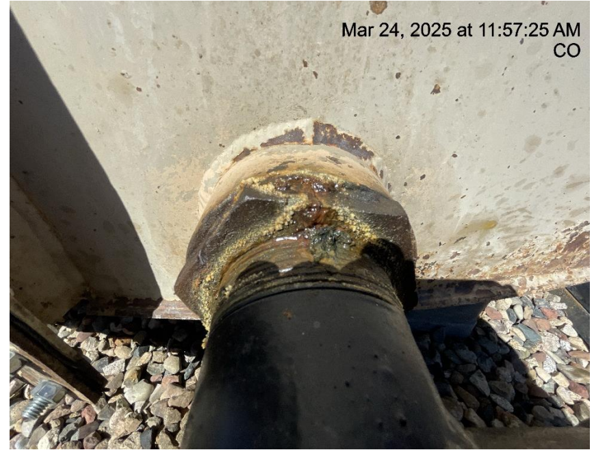
Photo # 6613 Mechanical Condition – Possible leak on tank valve
