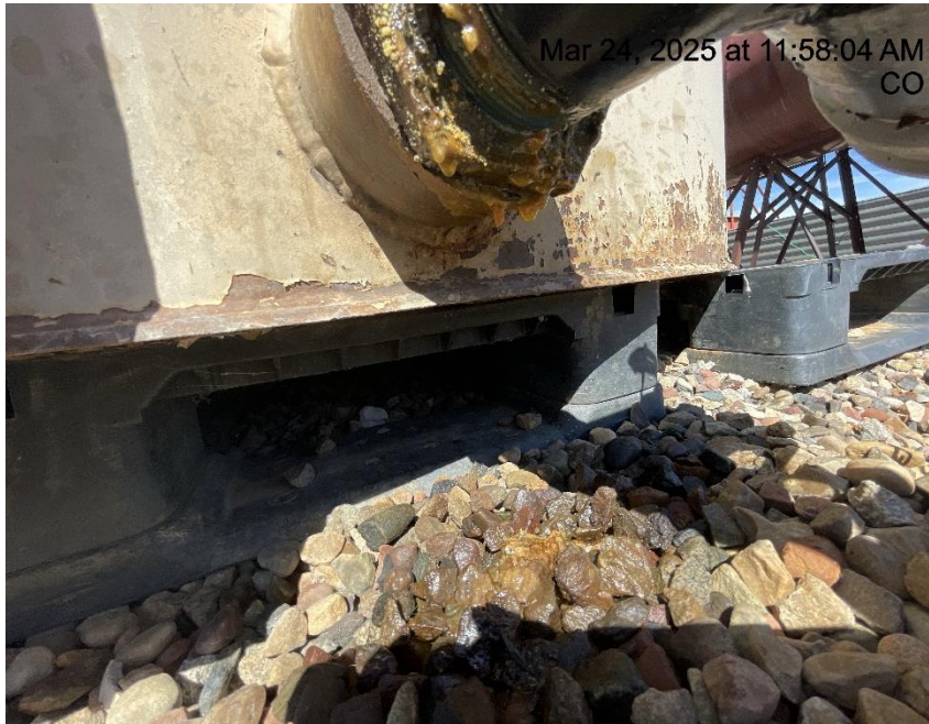
Photo # 6614 Mechanical Condition – Possible leak on tank valve
