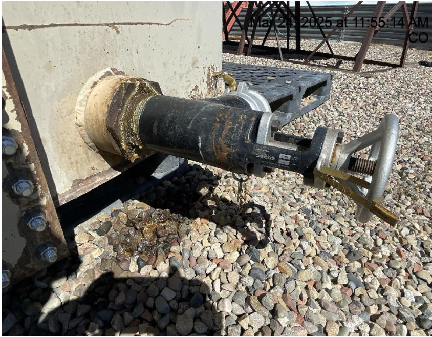
Photo # 6612 Mechanical Condition – Possible leak on tank valve
