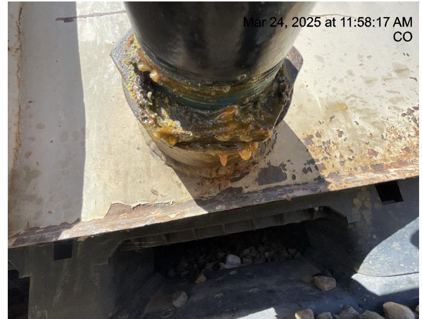
Photo # 6615 Mechanical Condition – Possible leak on tank valve
