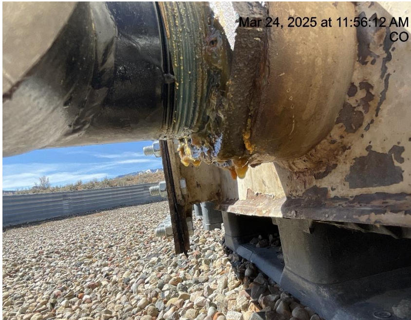
Photo # 6616 Mechanical Condition – Possible leak on tank valve
