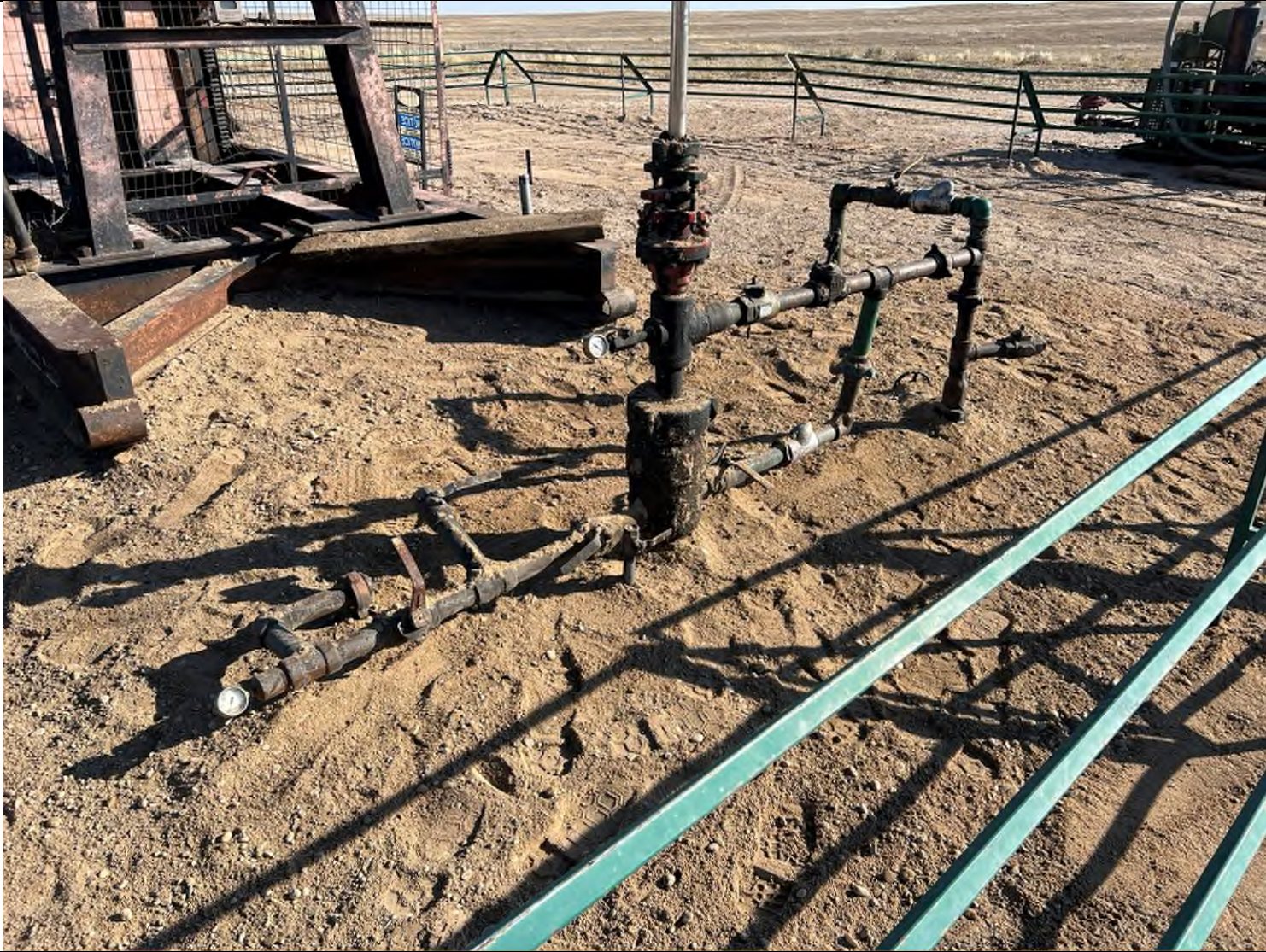
Description: Backfill around the wellhead
