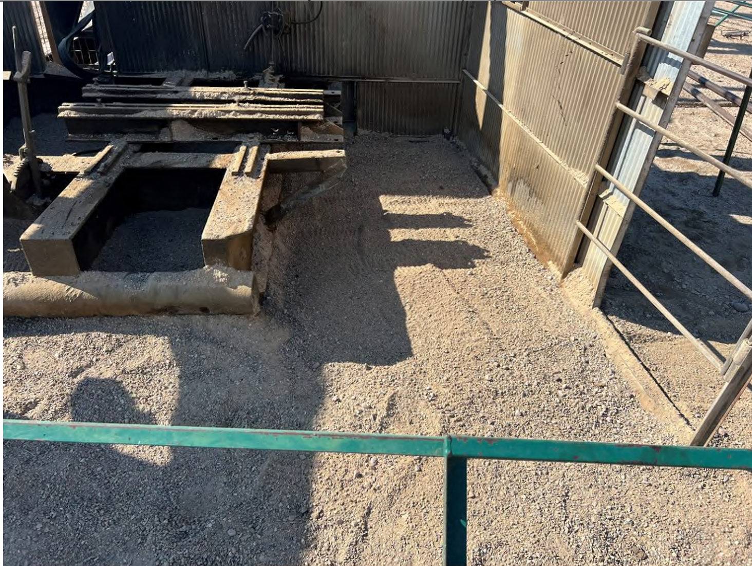
Description: Backfill below pump
