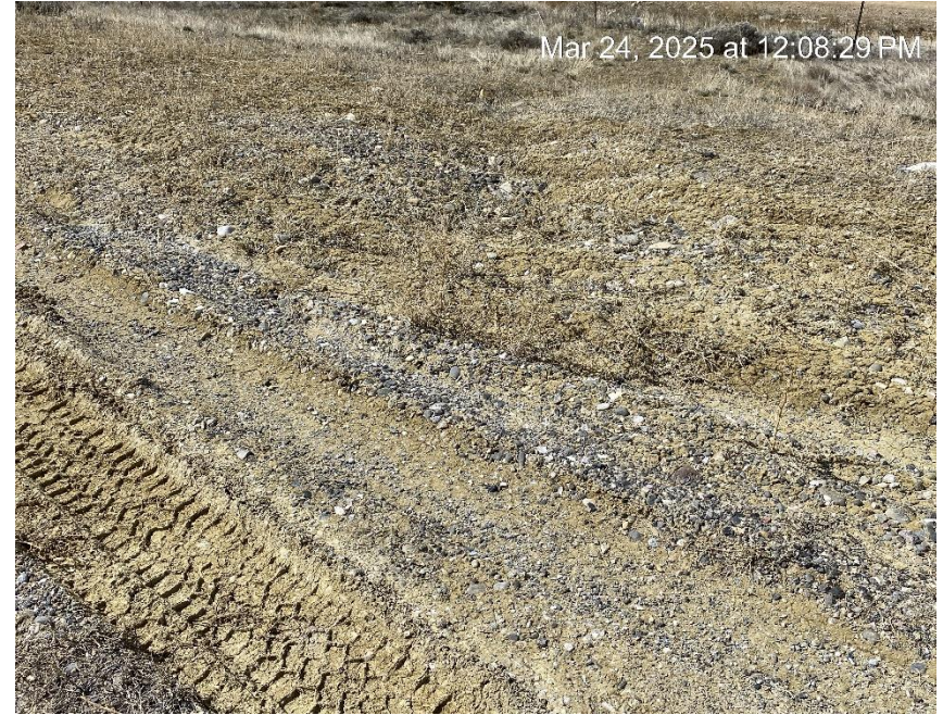
Erosion and sediment migration
