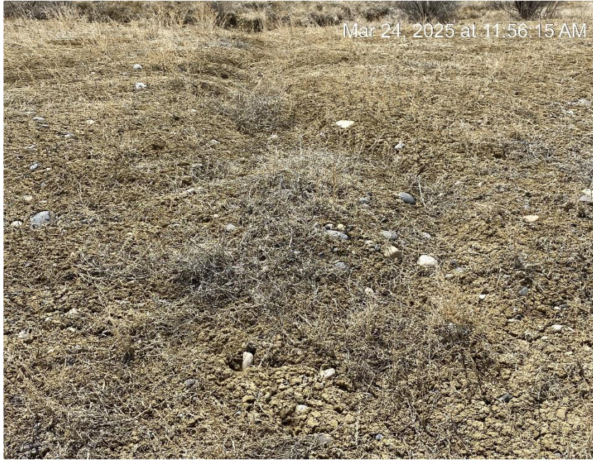
Erosion and sediment migration
