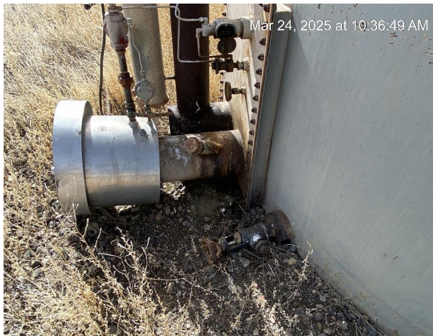
Leaking equipment and oily waste
