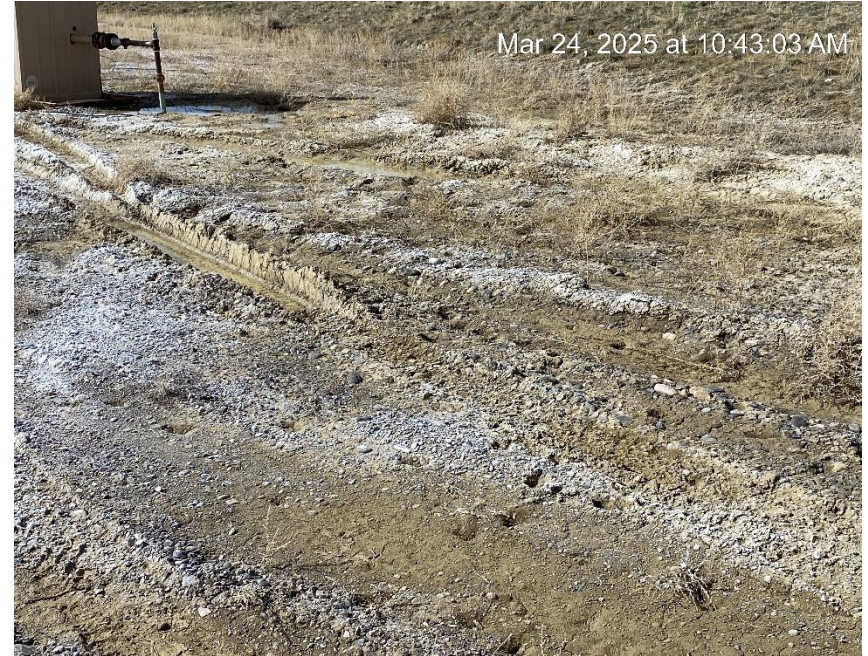
Stormwater BMPs not maintained
