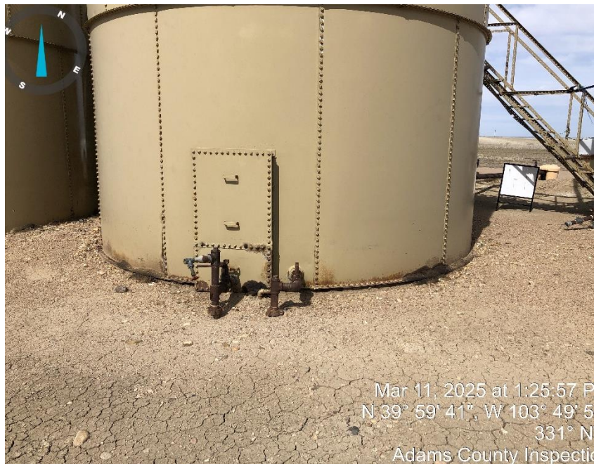
Photo #2 Some rusting & stained soil around tanks.
