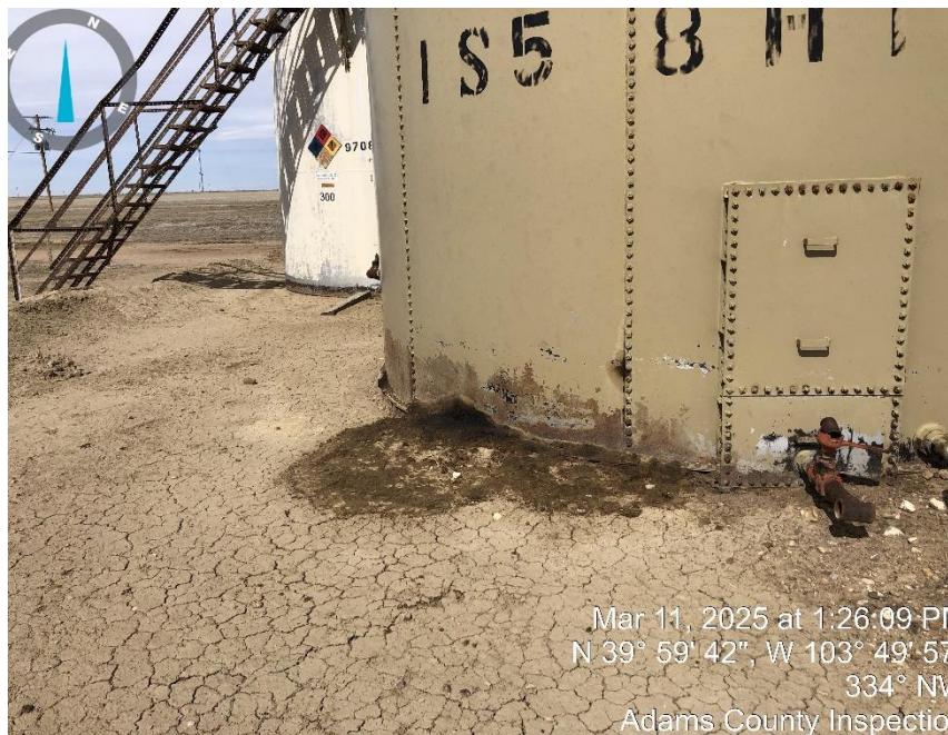
Photo #3 Some rusting & stained soil around tanks.
