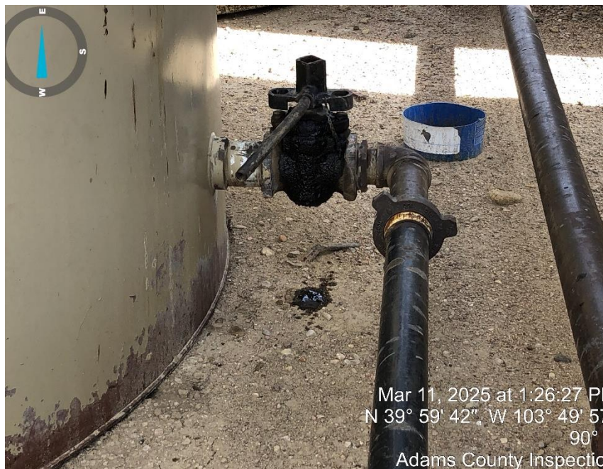
Photo #4 stained soil under valve
