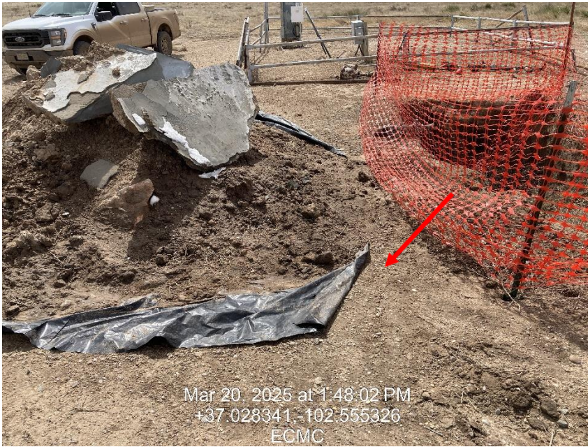
Photo 5 – Spoil Pile on liner, no berm, materials are migrating due to stormwater impacts
