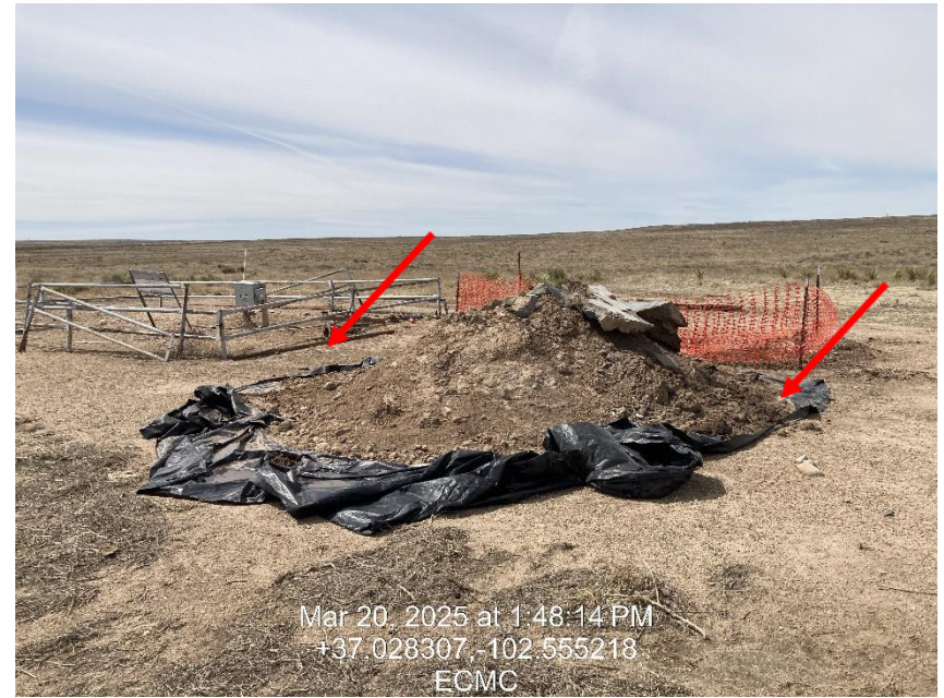
Photo 6 – Spoil Pile on liner, no berm, materials are migrating due to stormwater impacts
