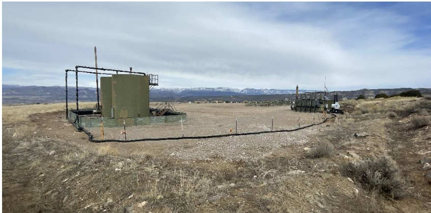
South West corner of location.
