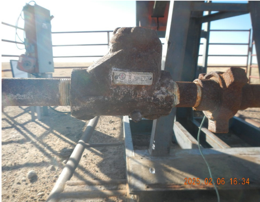
7. View of leaking check valve. Note salt staining on check valve body as seen 02/06/2025.
