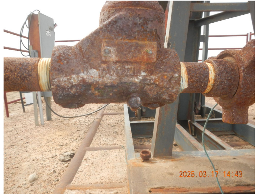
8. View of leaking check valve. Note salt staining on check valve body as seen 03/17/2025.
