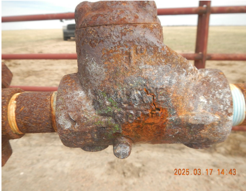
9. View of leaking check valve. Note salt staining on check valve body as seen 03/17/2025.
