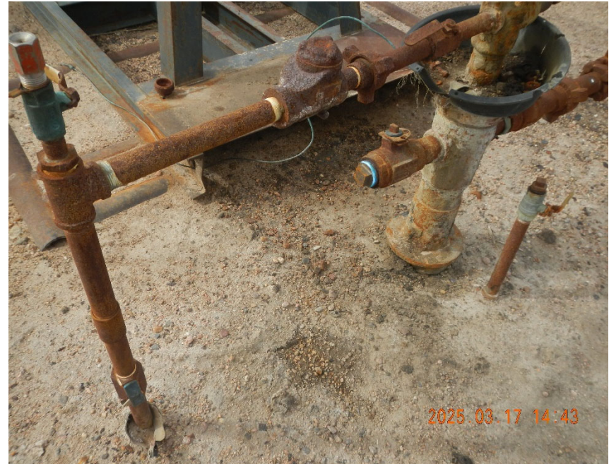
6. View of release location at wellhead. Note absence of fine sand at release point as seen 03/17/2025.
