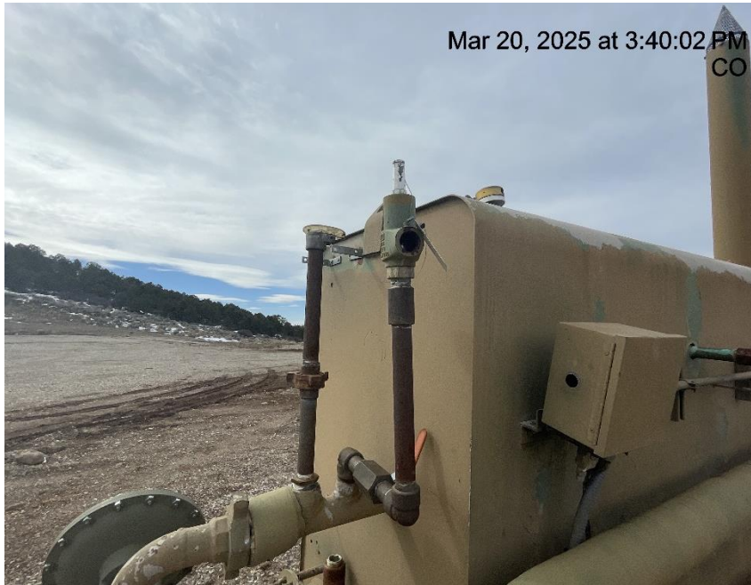
Photo # 6368 PRV vent line on separator does not comply with CECMC pressure safety device rules
