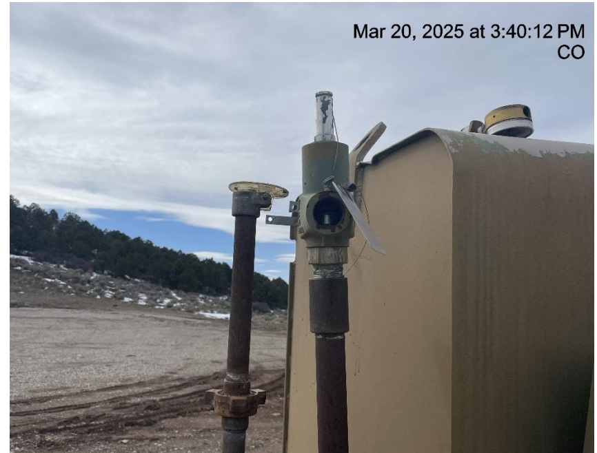
Photo # 6369 PRV vent line on separator does not comply with CECMC pressure safety device rules
