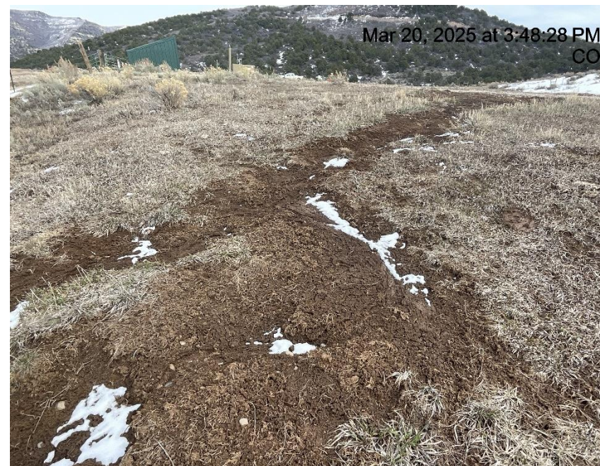
Photo # 6372 Erosion & transport of sediment off location /insufficient BMP's
