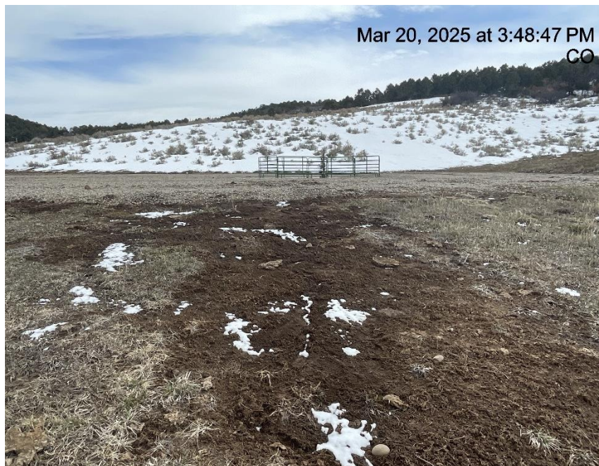
Photo # 6375 Erosion & transport of sediment off location /insufficient BMP's
