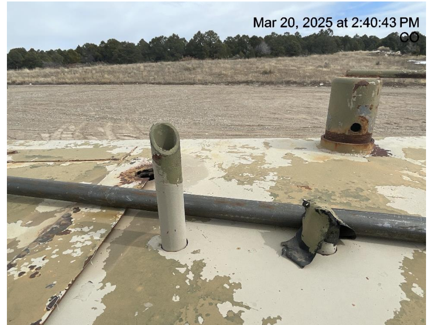
Photo # 6183 PRV vent line on separator does not comply with CECMC pressure safety device rules
