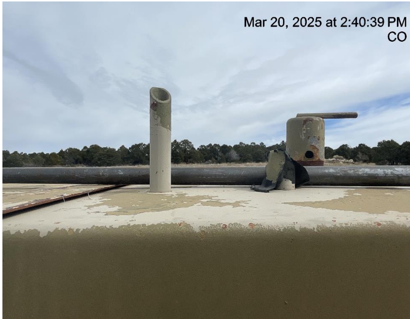
Photo # 6182 PRV vent line on separator does not comply with CECMC pressure safety device rules
