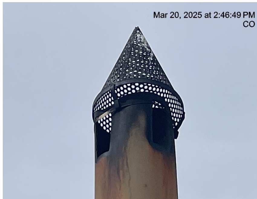
Photo # 6184 Bird protection on separator insufficient /burner stack available for entry by wildlife/wildlife hazard
