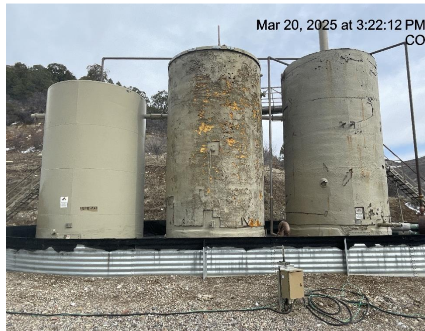
Photo # 6256 Middle tank lacks required labeling
