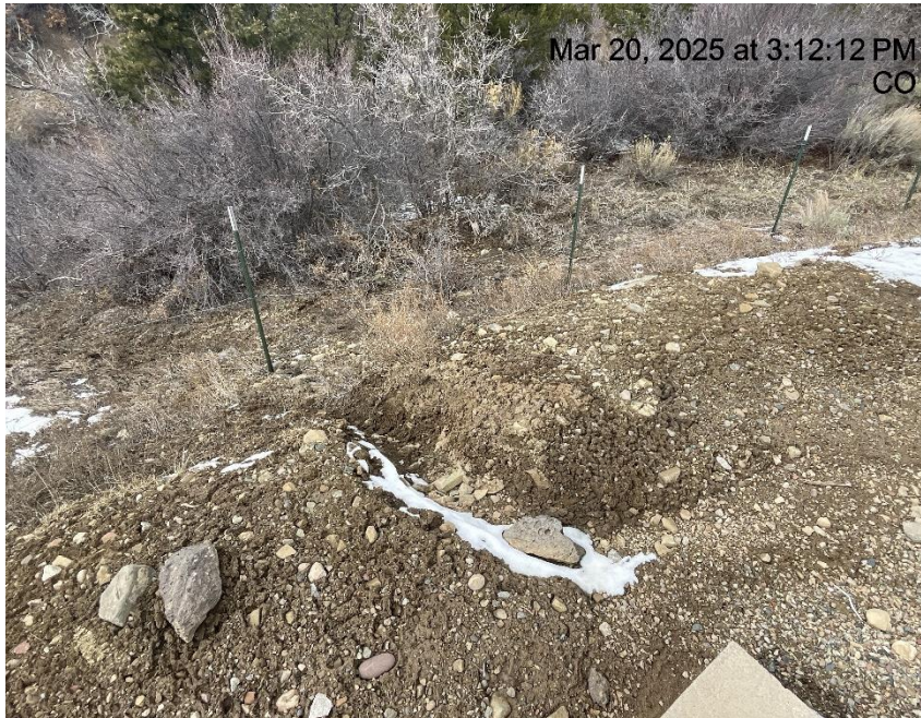
Photo # 6262 Erosion & transport of sediment off location /berm needs maintenance
