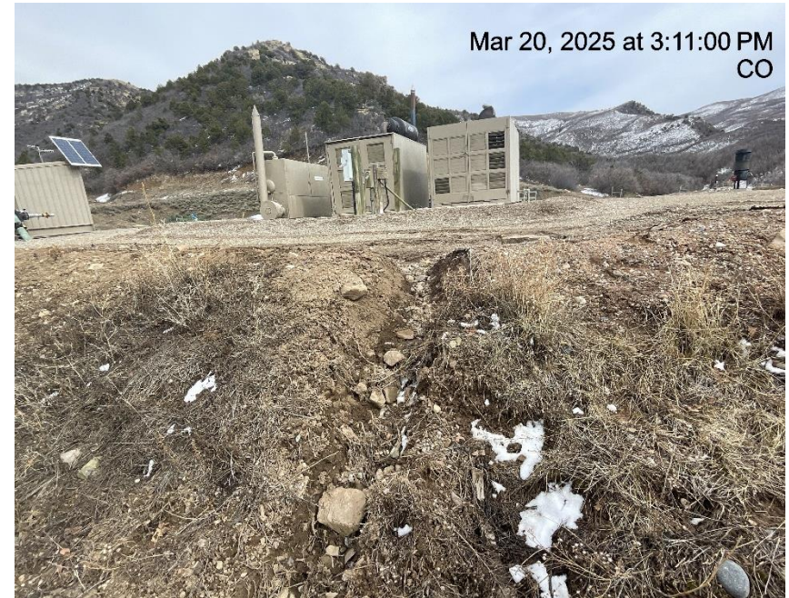
Photo # 6261 Erosion & transport of sediment off location /berm needs maintenance
