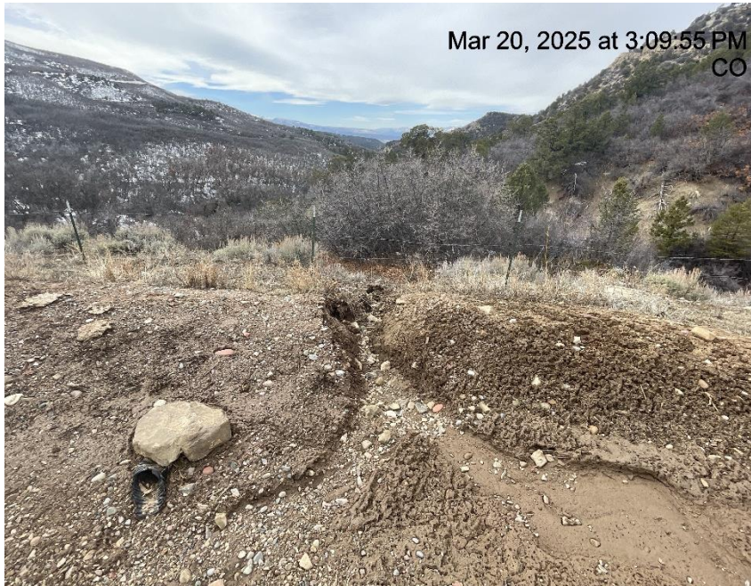
Photo # 6258 Erosion & transport of sediment off location /berm needs maintenance
