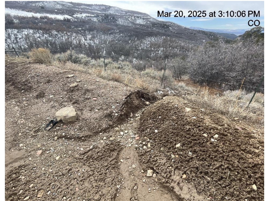
Photo # 6259 Erosion & transport of sediment off location /berm needs maintenance
