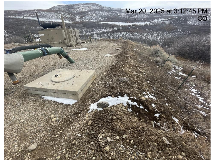
Photo # 6263 Erosion & transport of sediment off location /berm needs maintenance
