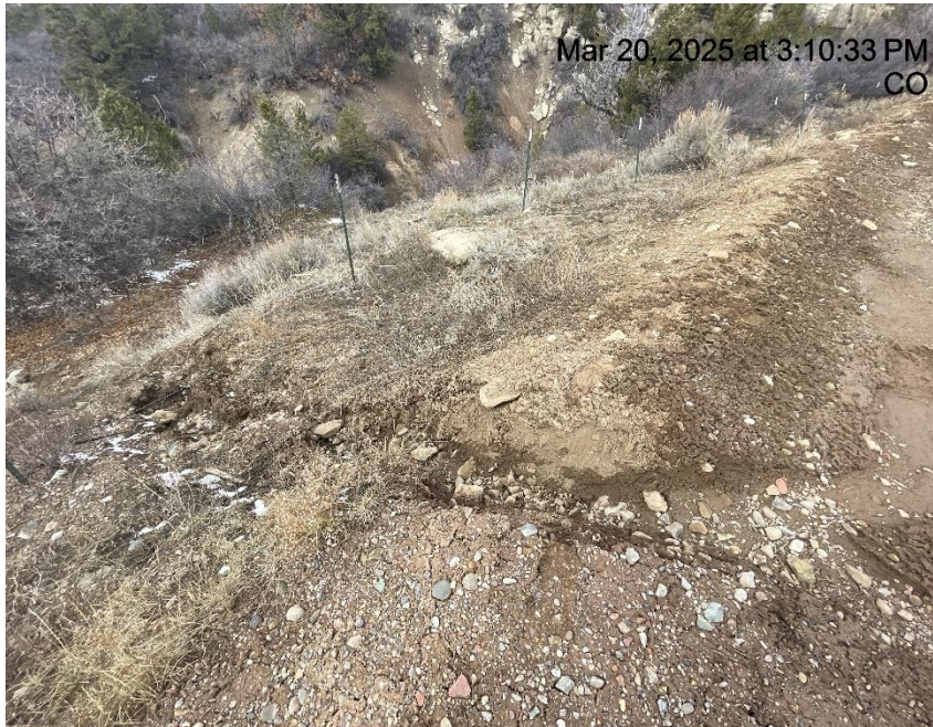
Photo # 6260 Erosion & transport of sediment off location /berm needs maintenance
