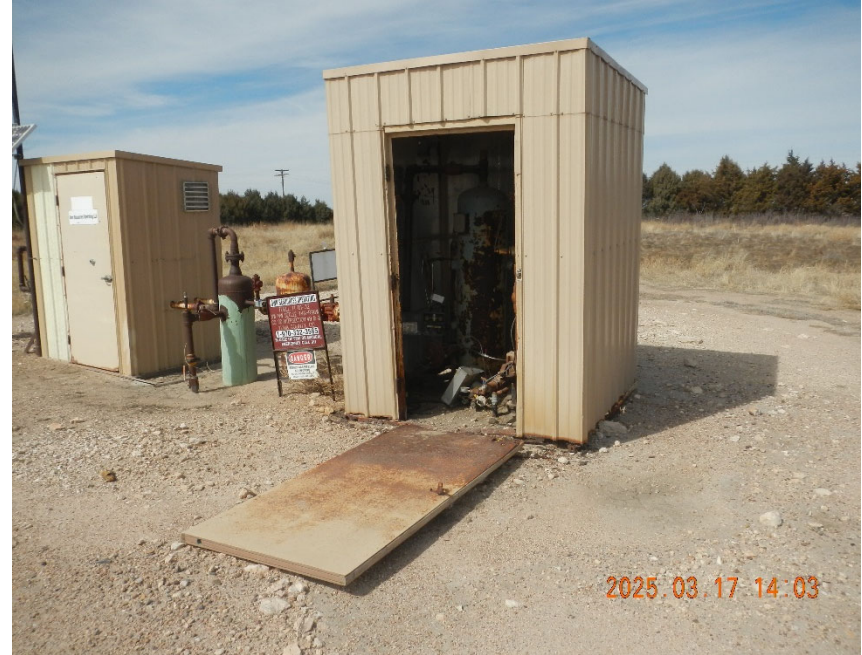
6. Separator/Well shed door 03/17/2025. Moved but not removed or repaired.
