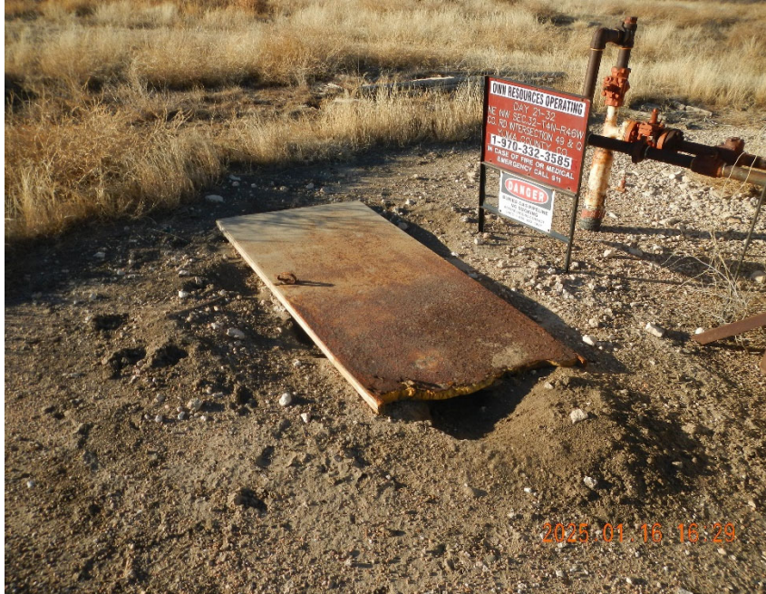
5. Separator/Well shed door 01/16/2025.
