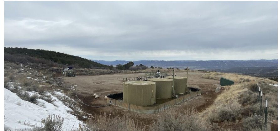
South East corner of location.
