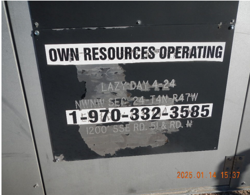
1. Lease sign at shared gas meter run on 01/14/2025.
