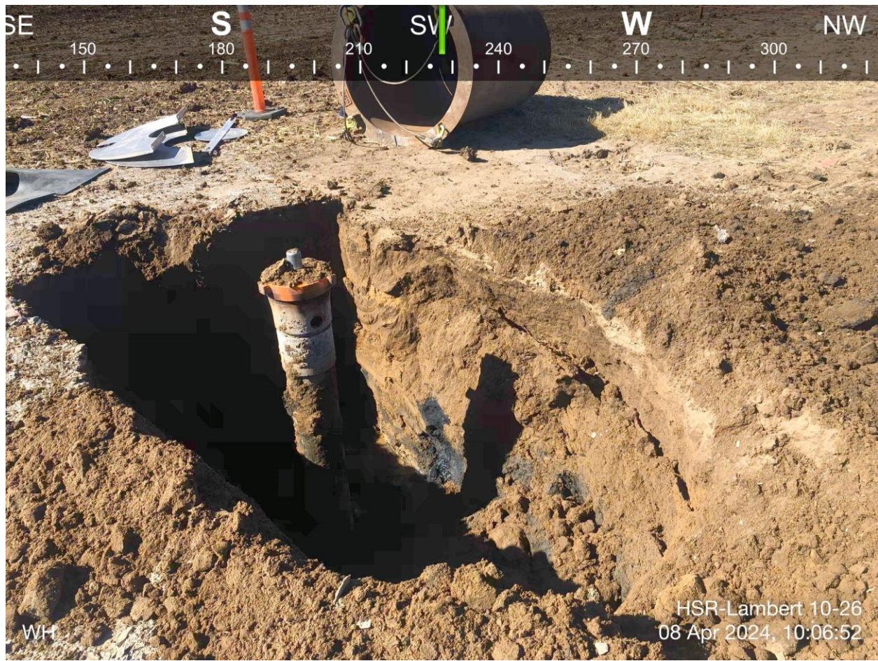
Initial Wellhead Decommissioning
