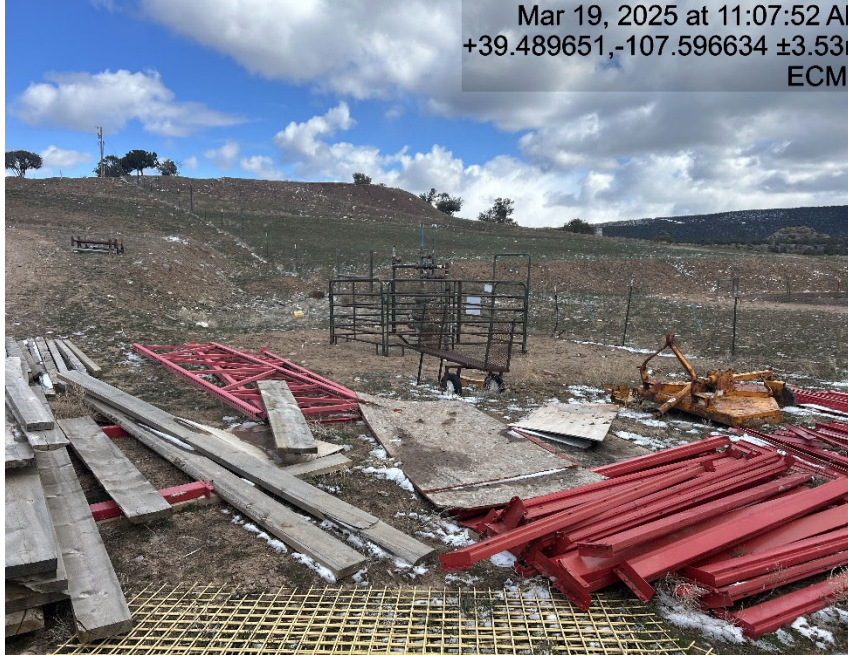
Stored materials around well head
