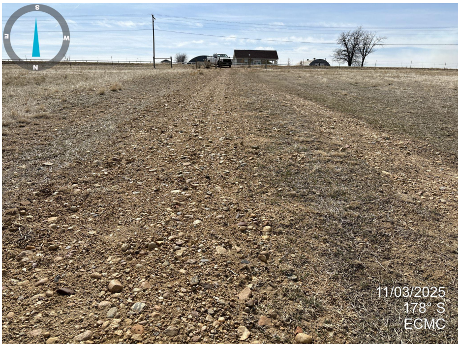
Photo 3. Looking south down access road. Gravel on the access road.
