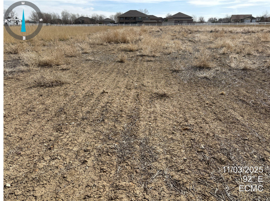
Photo 2. Looking east across the tank battery. It appears that reclamation has been conducted with evidence of straw. There are large patches of bare soil with no desirable vegetation establishment.
