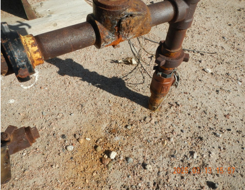
3. View of water line on wellhead tree with damp stained soil below check valve.
