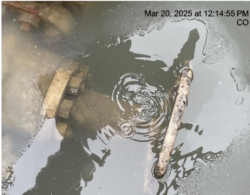
Photo # 5665 Mechanical Condition - Possible leak on CSF 42B-07-07-91 wellhead casing valve
