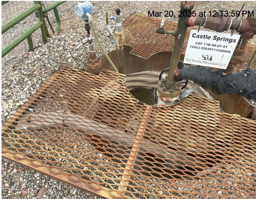
Photo # 5669 Wildlife egress board improperly placed/cellar cover has rendered egress board unusable
