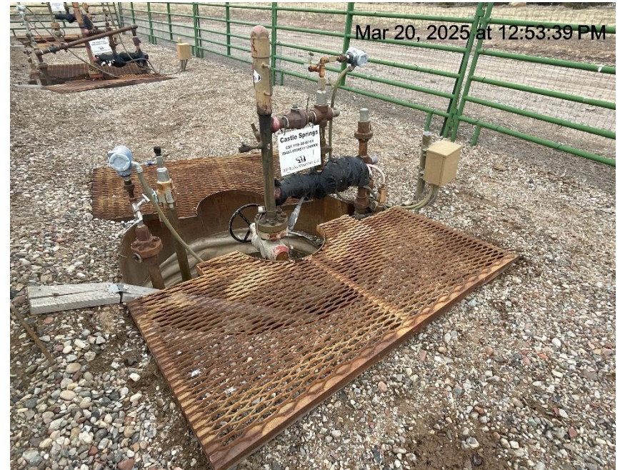
Photo # 5670 Egress board adjusted by TEP lease operator during inspection
