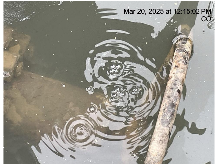
Photo # 5666 Mechanical Condition - Possible leak on CSF 42B-07-07-91 wellhead casing valve
