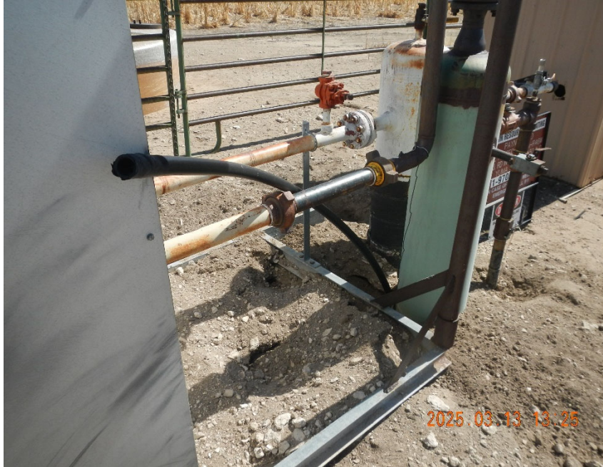
5. Open ended poly line at metering location.
