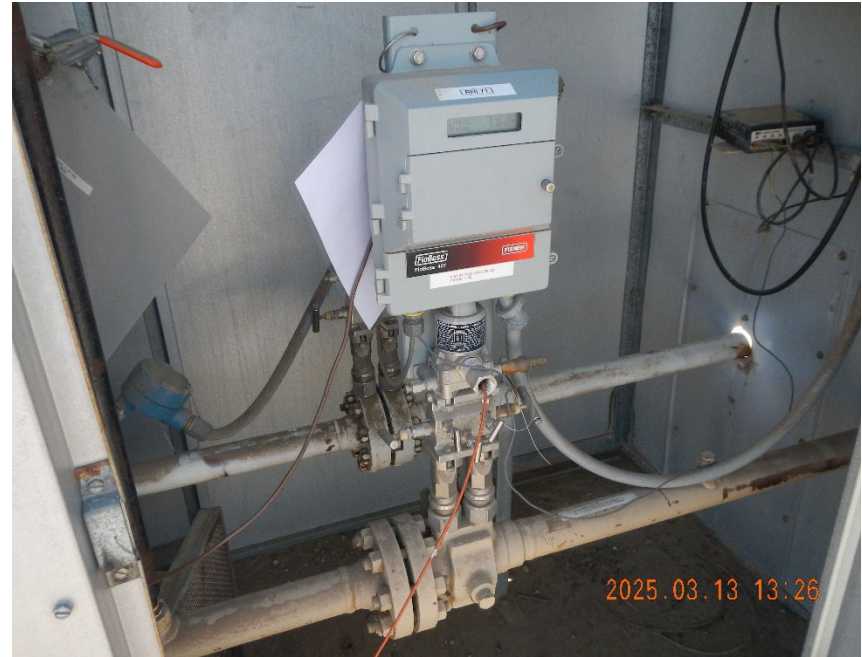
4. Gas meter inside meter shed.
