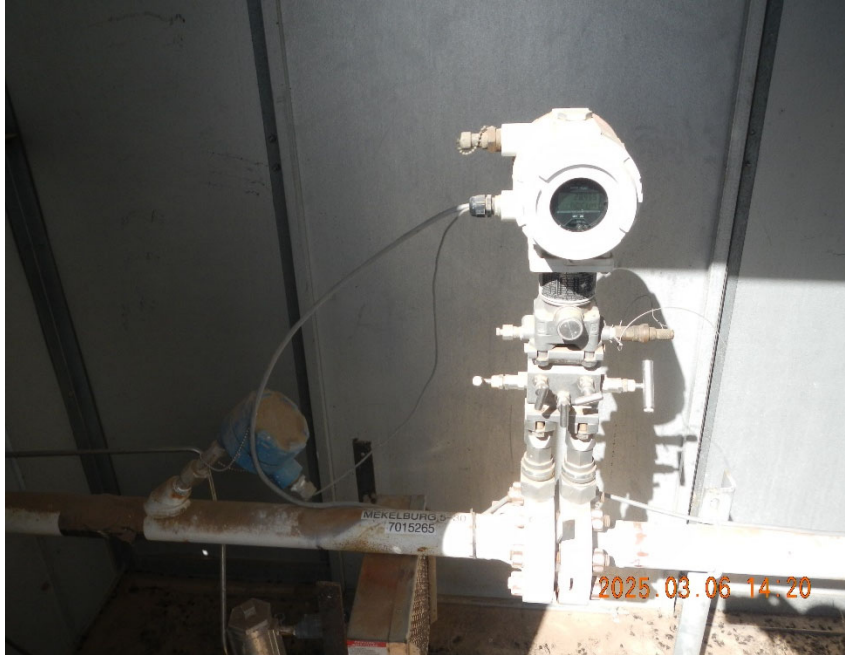
3. Gas meter inside meter shed.
