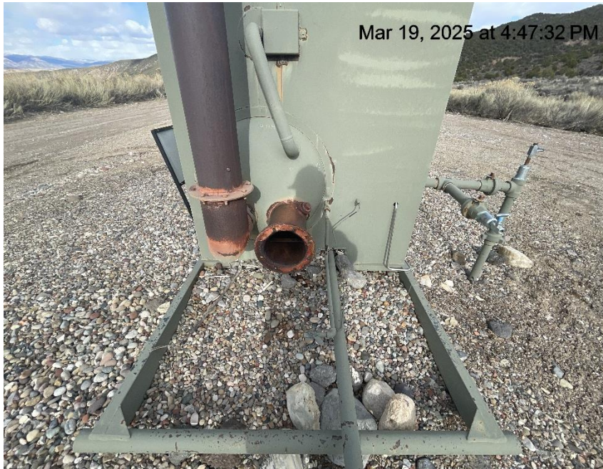
Photo # 5607 Burner assembly open ended/wildlife hazard /available for entry by wildlife
