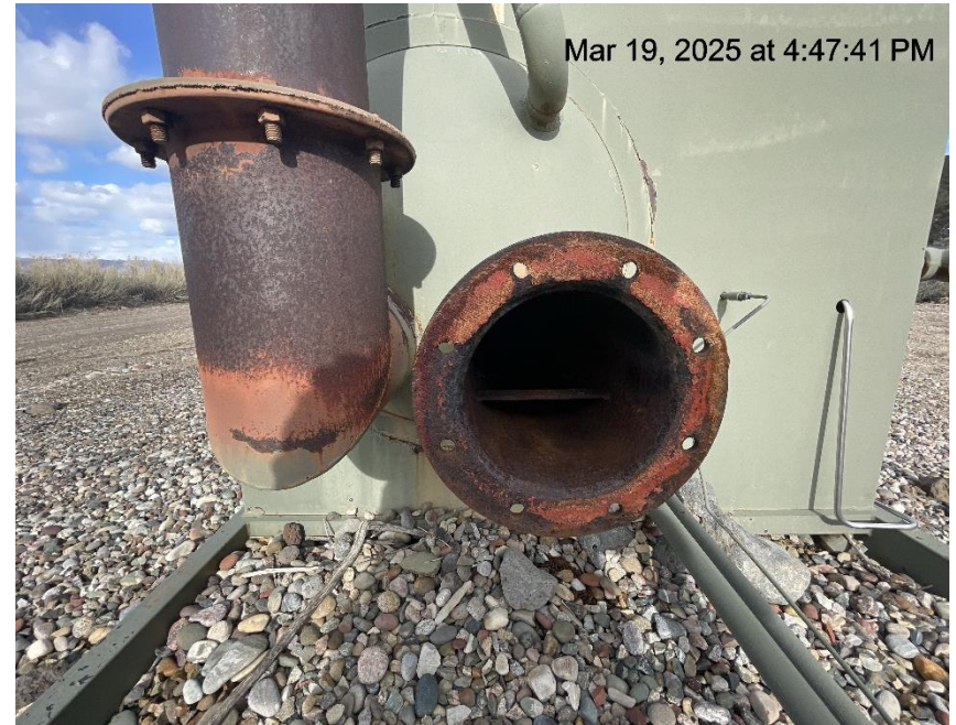
Photo # 5608 Burner assembly open ended/wildlife hazard /available for entry by wildlife
