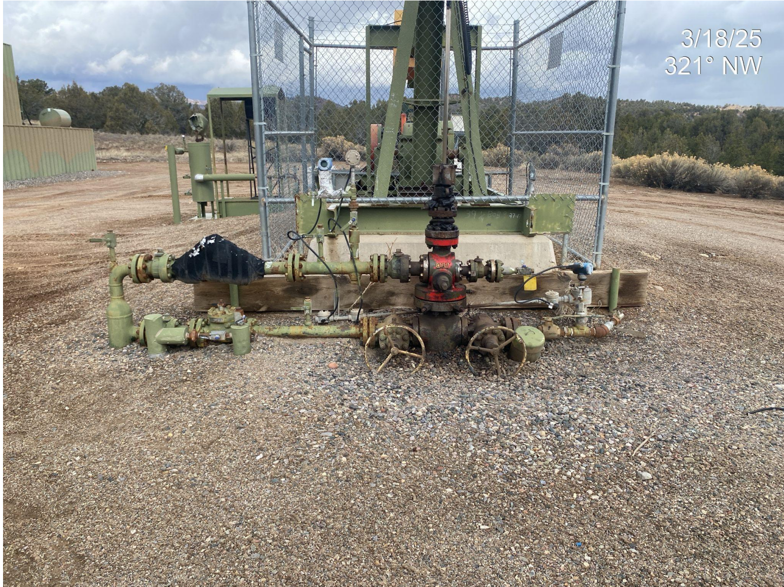
Photo 3. Stained soils/gravel at wellhead have been removed.
