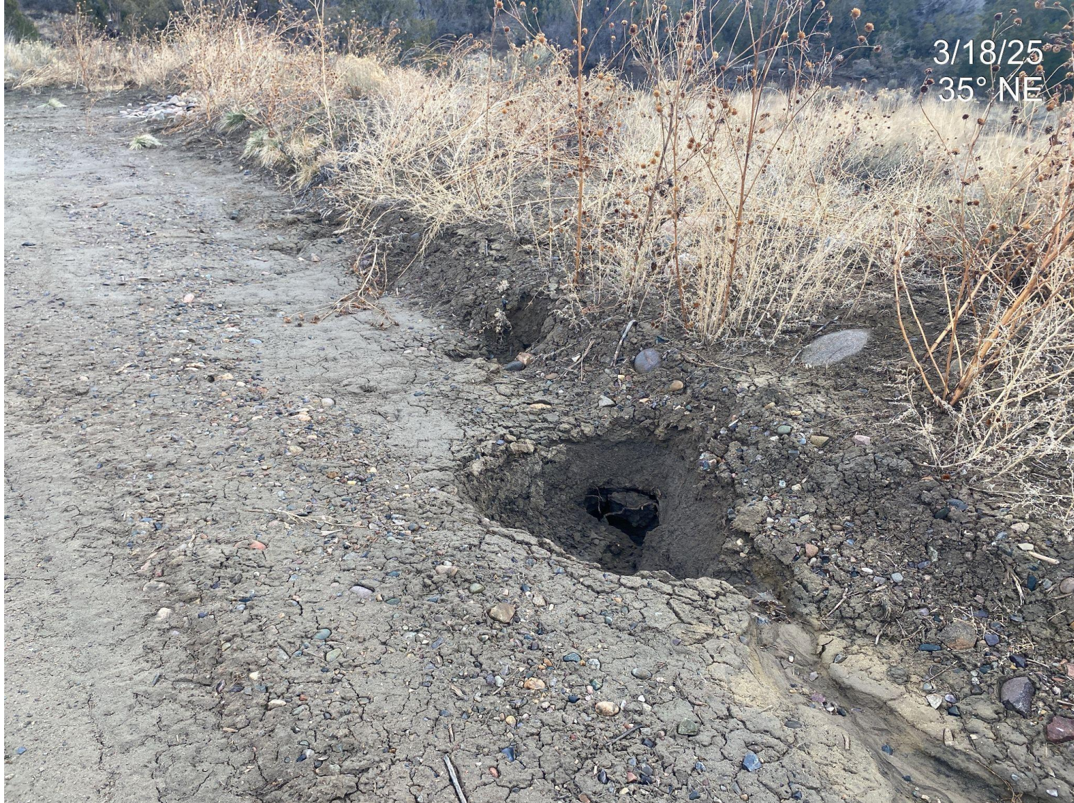
Photo 4. Hole/erosion tunnel forming along the eastern perimeter berm.
