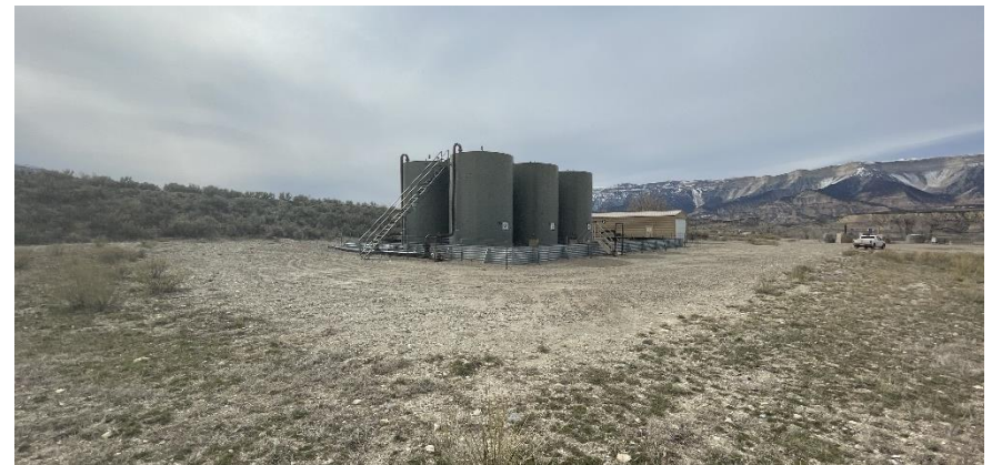
South East corner of location.
