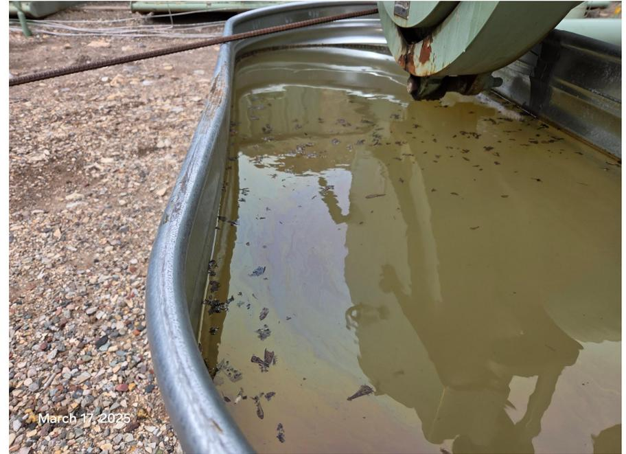
**Photo 3:** Photos taken from the pipeline equipment on the southeast end of the Location. Photo shows containment measure has filled with fluid, and a chemical sheen is apparent. Photo also shows wildlife protection measures are missing or insufficient.
