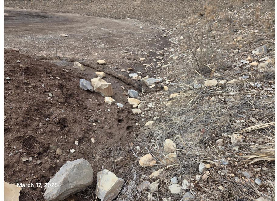
**Photo 8:** Continued from photo 7. Photo shows erosion log placed at the soil stockpile has been crushed, and is no longer in proper functioning condition to minimize sediment migration for the stockpile. Photo also shows soil stockpile has been placed within areas of the perimeter stormwater diversion ditch.
