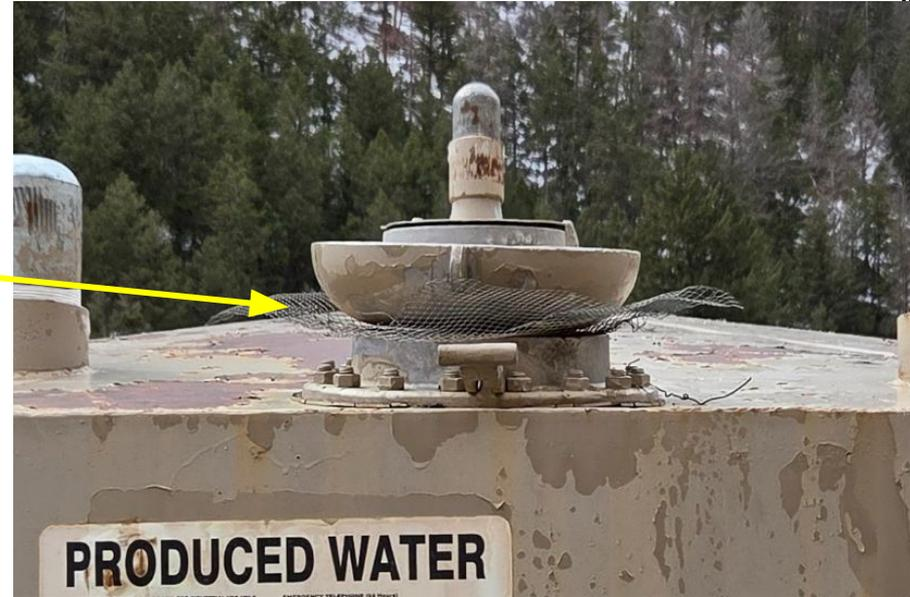
**Photo 4:** Photos taken from the produced water tank on the east end of the Location. Photo shows tank hatch is broken; Operator appears to have taken the top portion of the hatch and placed it upside down over the opening. Tank is improperly closed to prevent emissions from venting.
