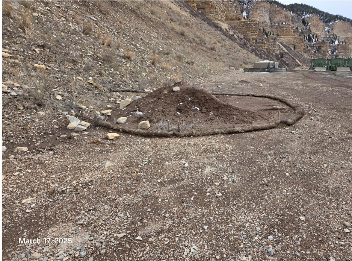
**Photo 7:** Photo taken from the northeast end of the working pad surface, facing southeast. Photo shows soil stockpile has been placed within areas of the perimeter stormwater diversion ditch- placement of stockpiles within a stormwater diversion ditch does not comport with stockpile protection requirements, and places the soils at risk to commingling with stormwater runoff, and sediment transport.
