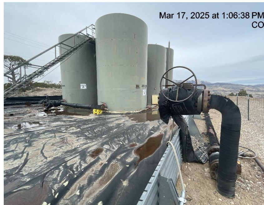
Photo # 4660 Piping disconnected & blind flanged
