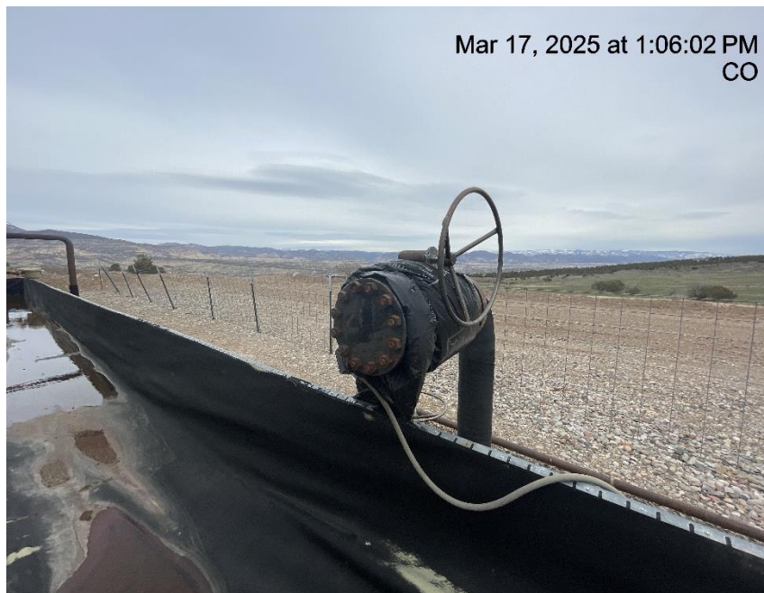
Photo # 4659 Piping disconnected & blind flanged
