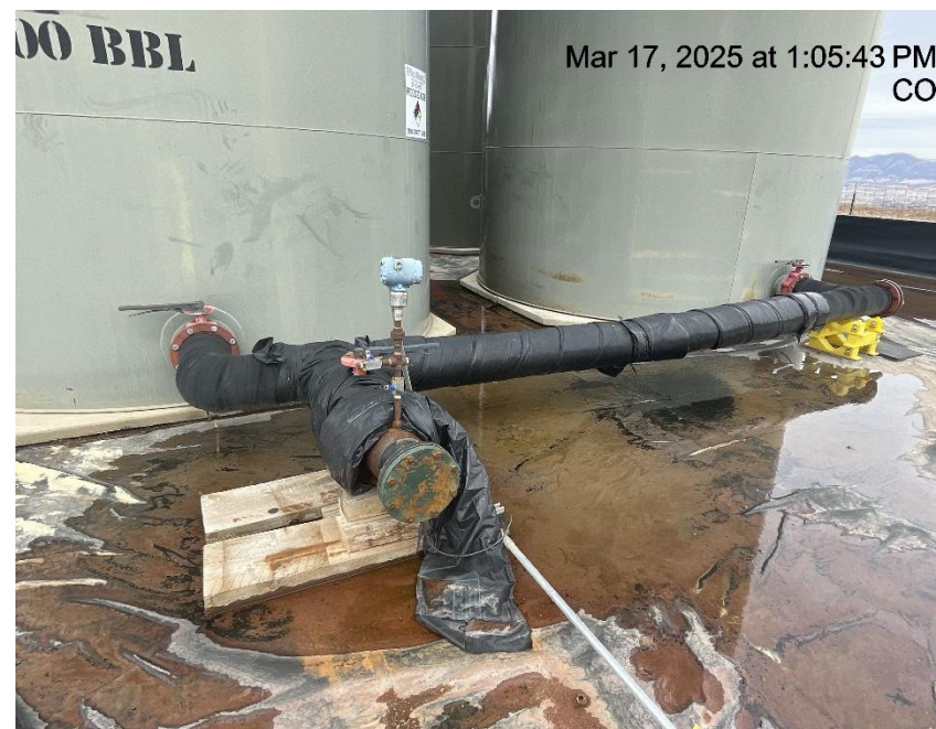
Photo # 4658 Piping disconnected & blind flanged
