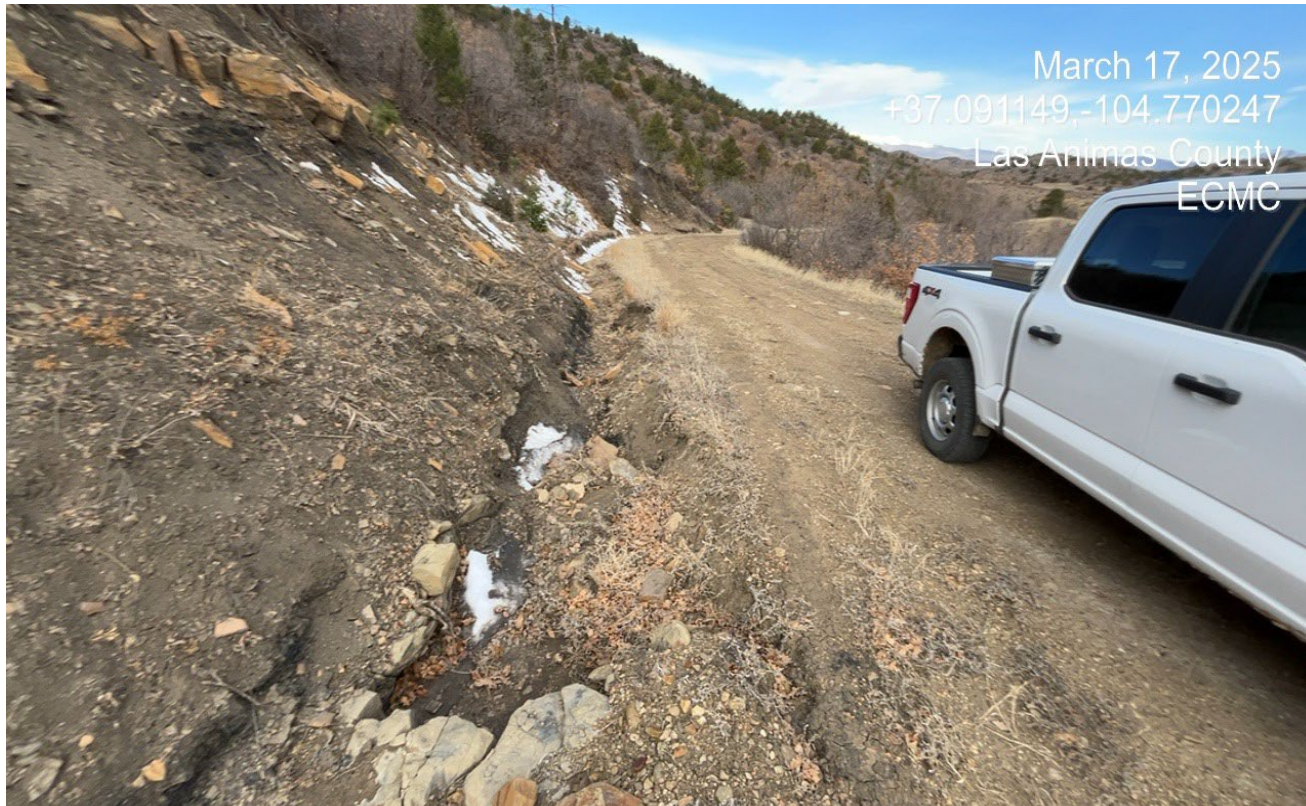
Photo 3. Facing west along the access road traveling east from the wellsite. This area along the road side has eroded and will need BMP's such as check dams, culverts, ect. to further prevent erosion.
