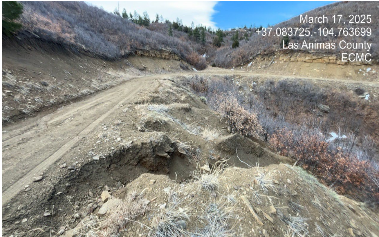
Photo 6. Facing back south at the same area as the previous photo. This area has eroded and will need to be repaired and stabilized.
