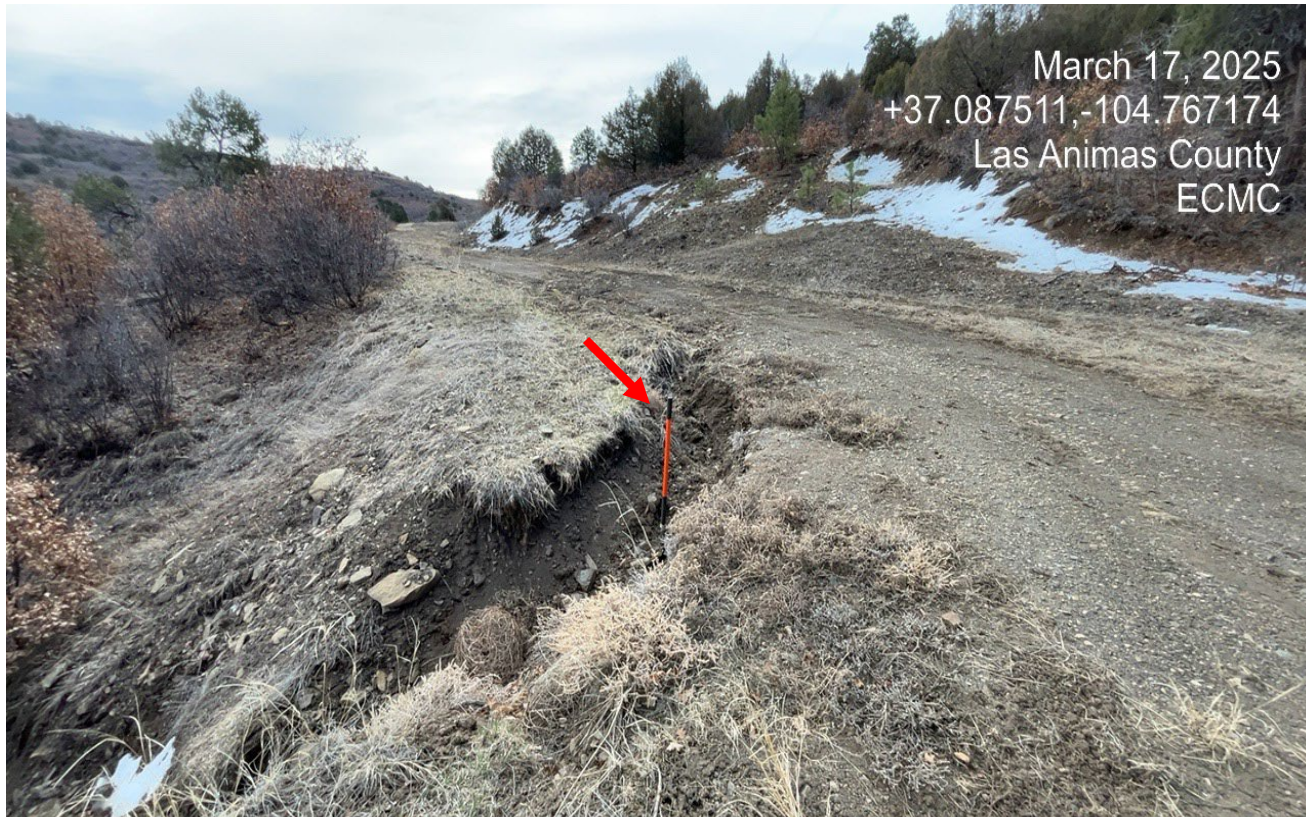
Photo 4. Facing east further along the road. This area has eroded and will need to be repaired and stabilized. Red arrow points to 4.5 ft shovel in the erosion gully.
