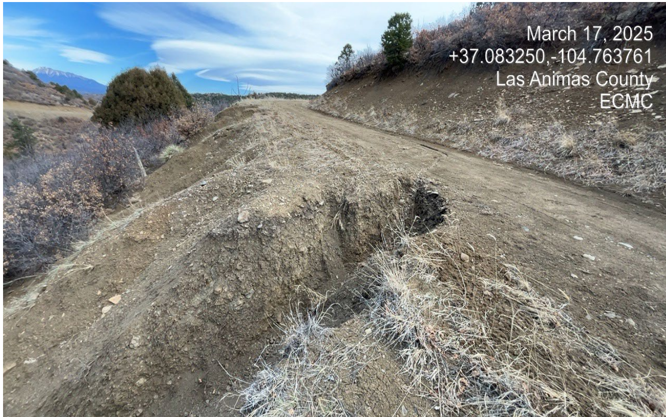
Photo 5. Facing north toward the fill slope of the road. This area has eroded and will need to be repaired and stabilized.
