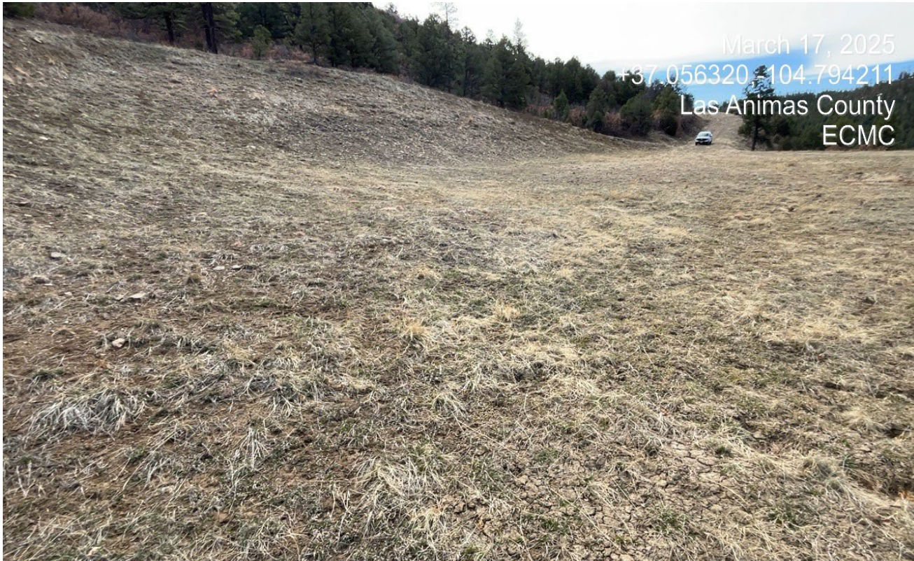
Photo 8. Facing southeast along the cut slope which is stabilized with perennial vegetation.
