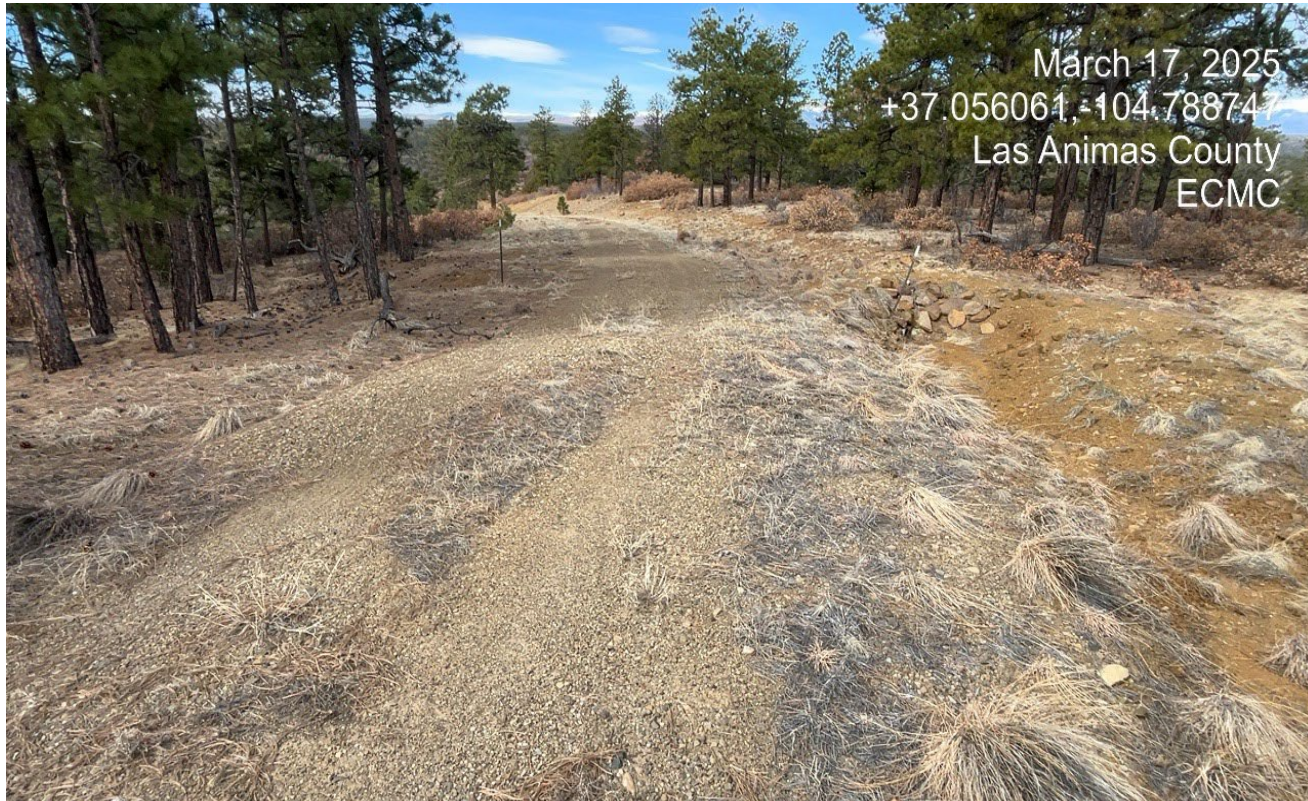
Photo 1. Facing west along the access road. BMP's are installed and in good condition along the road.
