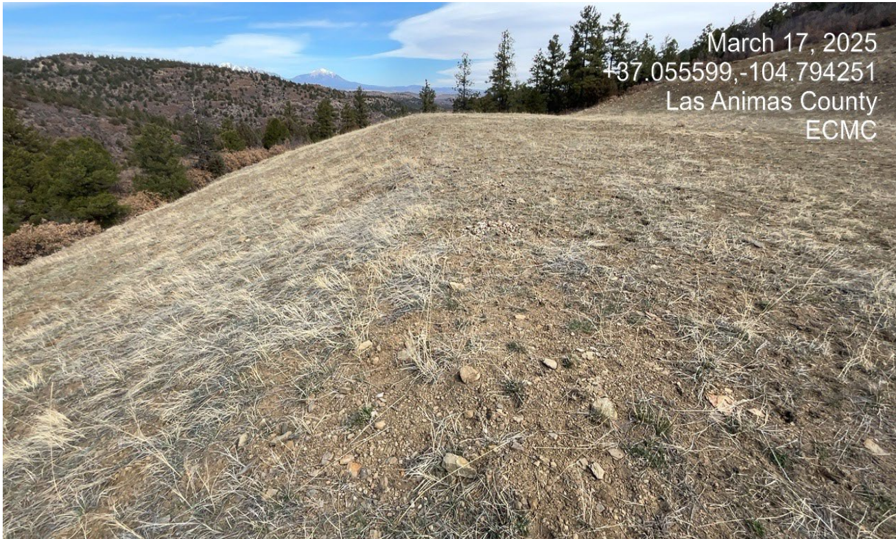
Photo 6. Facing west along the fil slope which is stabilized with perennial vegetation.
