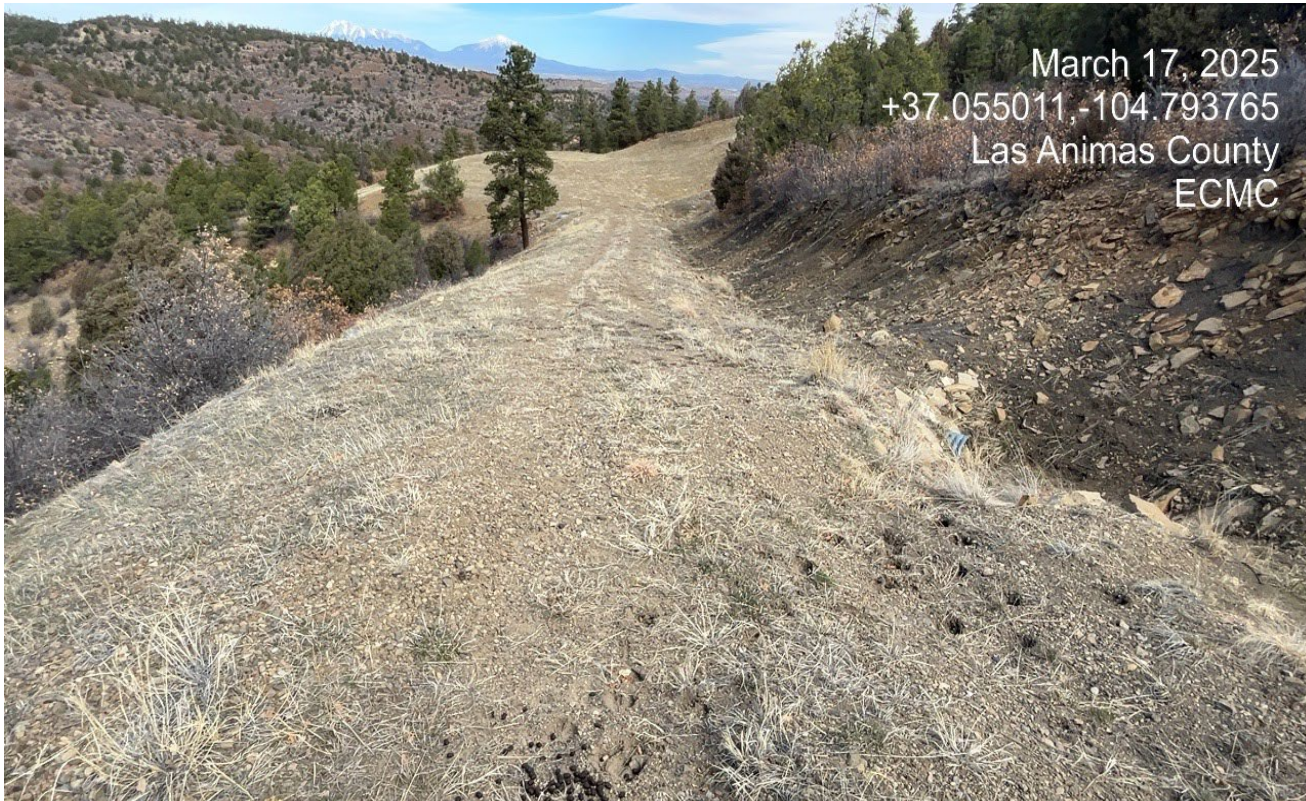
Photo 4. Facing north along the access road toward the location.
