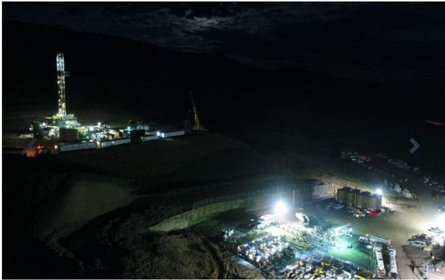
Photo 1. Drilling at Laramie's 24-7 well pad (left) and completions & flowback operations at Laramie's 24-6A well pad (right).
