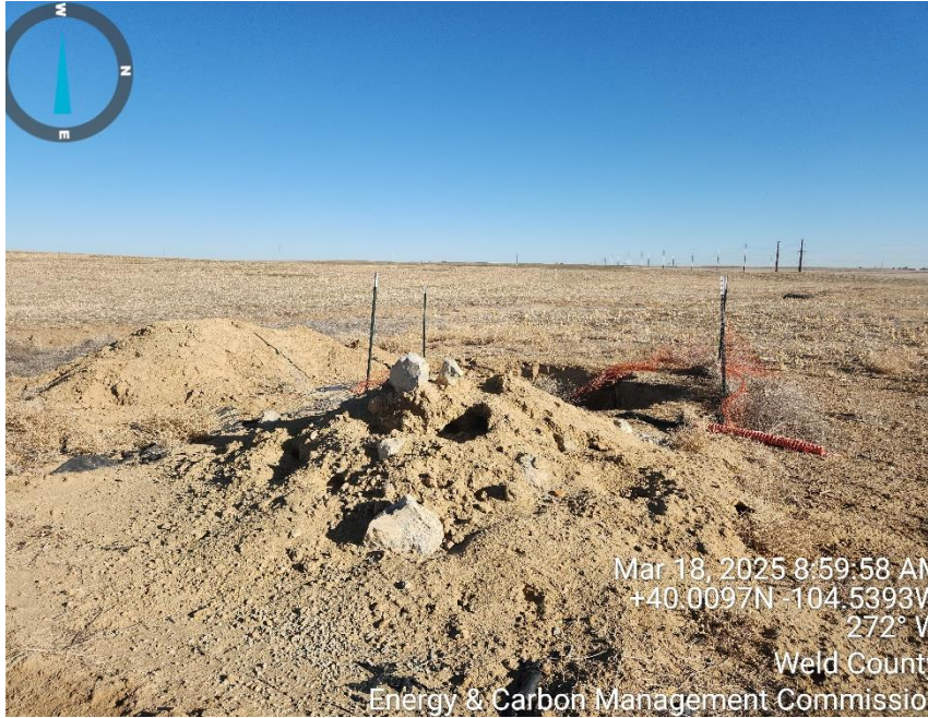
Photo 1 well head site
