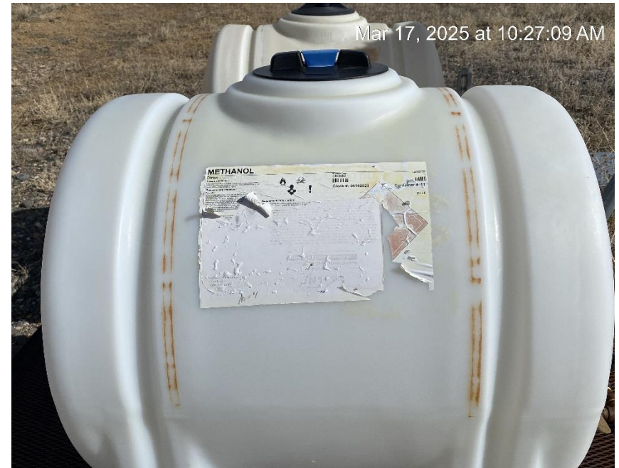
Inadequate tank label
