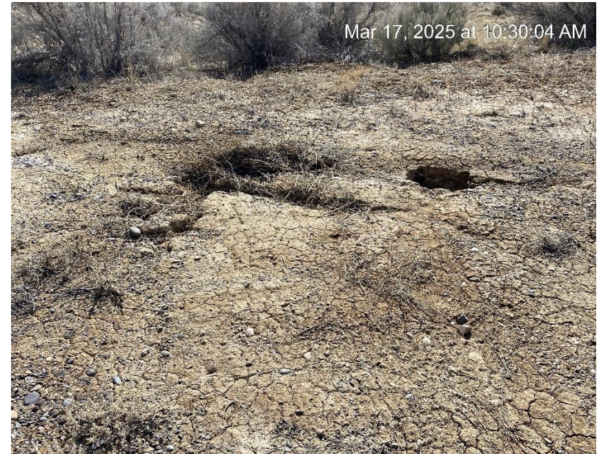
Lack of Stormwater BMP maintenance
