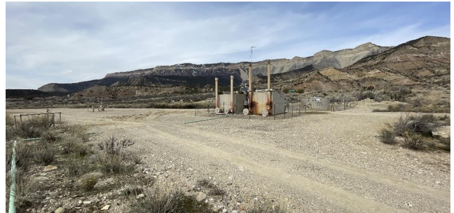
South East corner of location.
