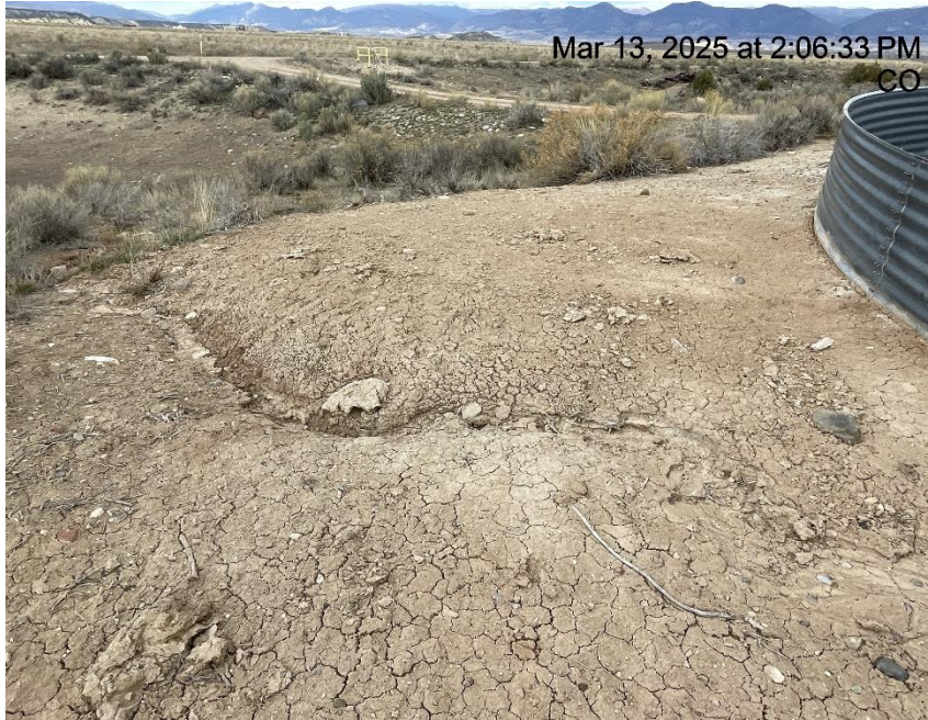
Photo # 3343 Erosion & transport of sediment off location /insufficient BMP's
