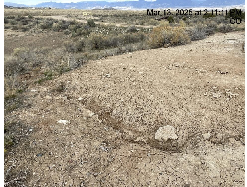
Photo # 3344 Erosion & transport of sediment off location /insufficient BMP's
