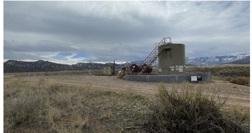
North East corner of location.
