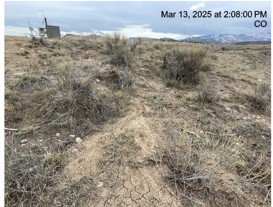
Photo # 3346 Erosion & transport of sediment off location /insufficient BMP's
