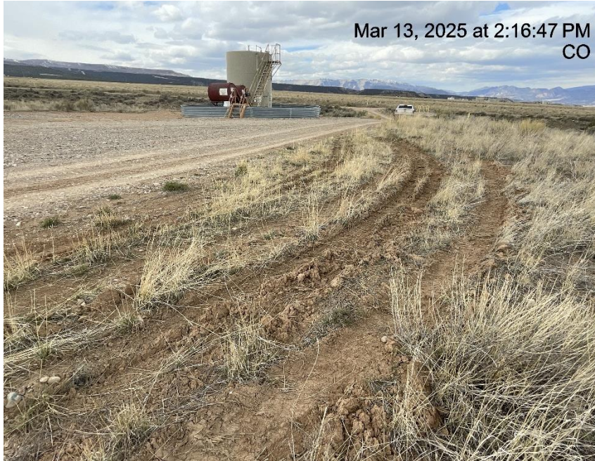
Photo # 3339 Failure to minimize surface disturbance
