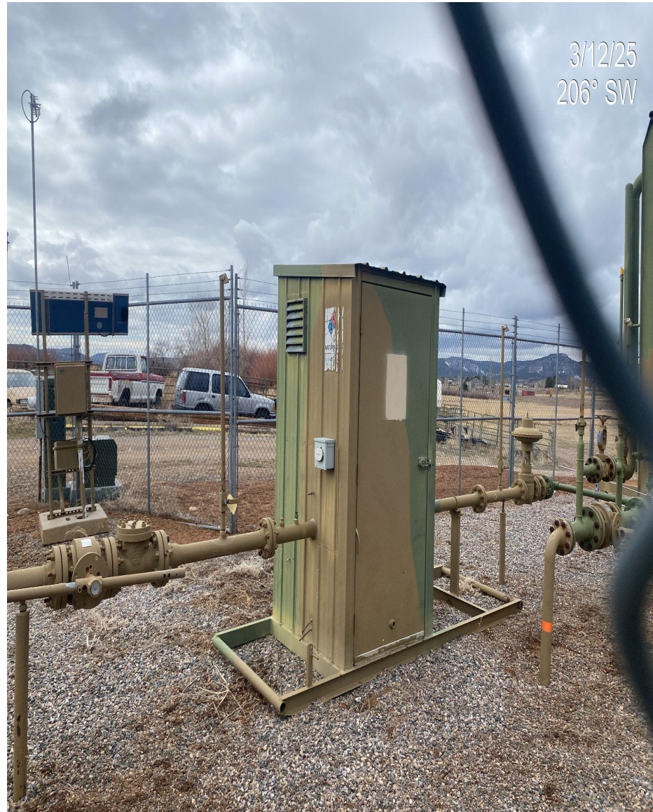
Photo 3. Separator equipment labels have deteriorated and are no longer legible.
