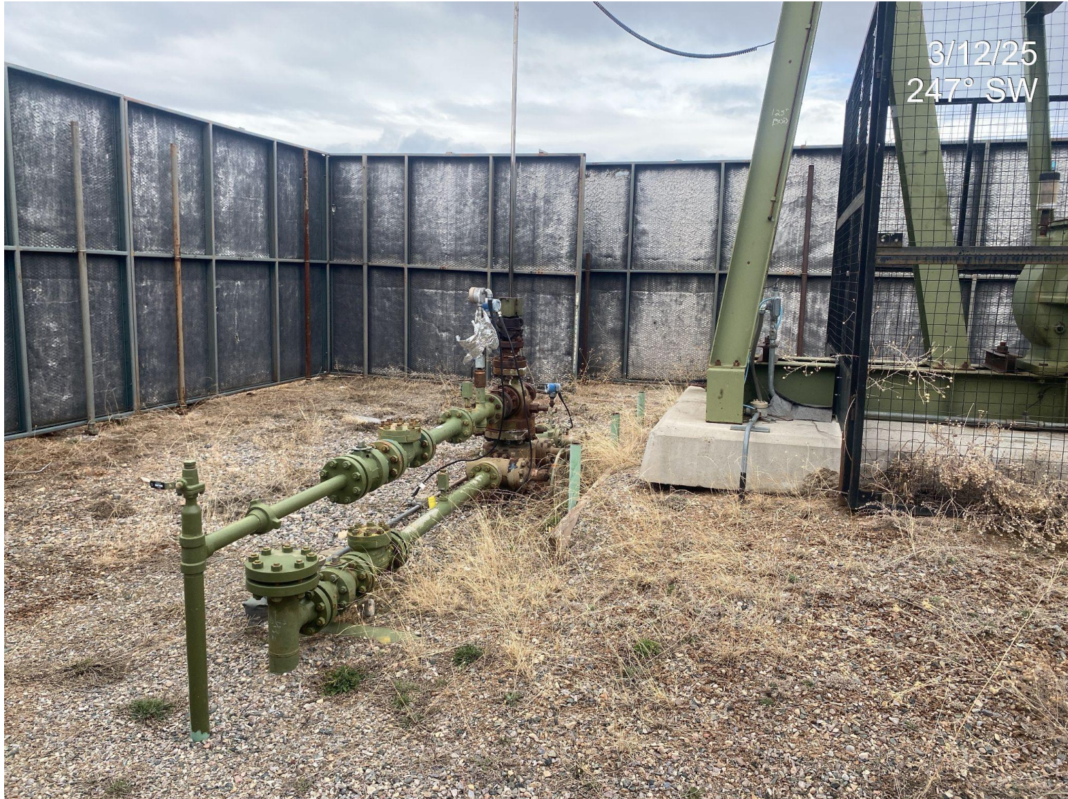
Photo 3. Stained soils at wellhead have been removed. Combustible material are encroaching on wellhead.
