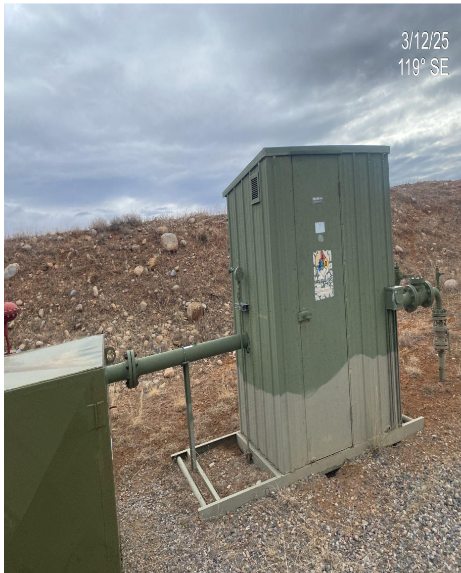
Photo 2. Labels at separators are deteriorating and no longer legible.
