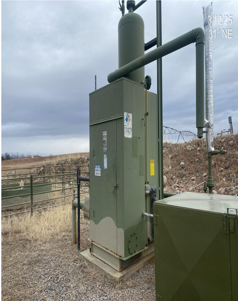
Photo 2. Labels at separators are deteriorating and no longer legible.
