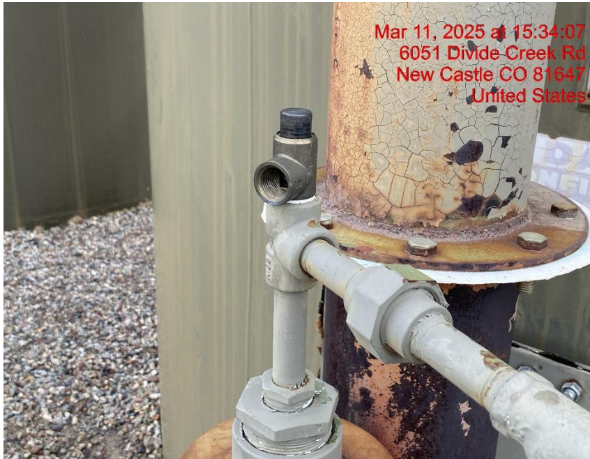
PRV Terminates in Unsafe Manner – Photo #07192
