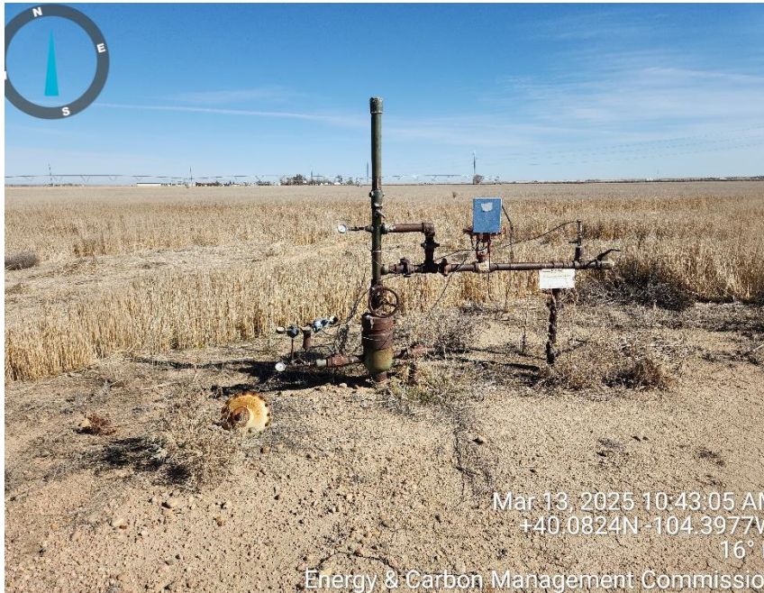
Photo 1 well head and equipment
