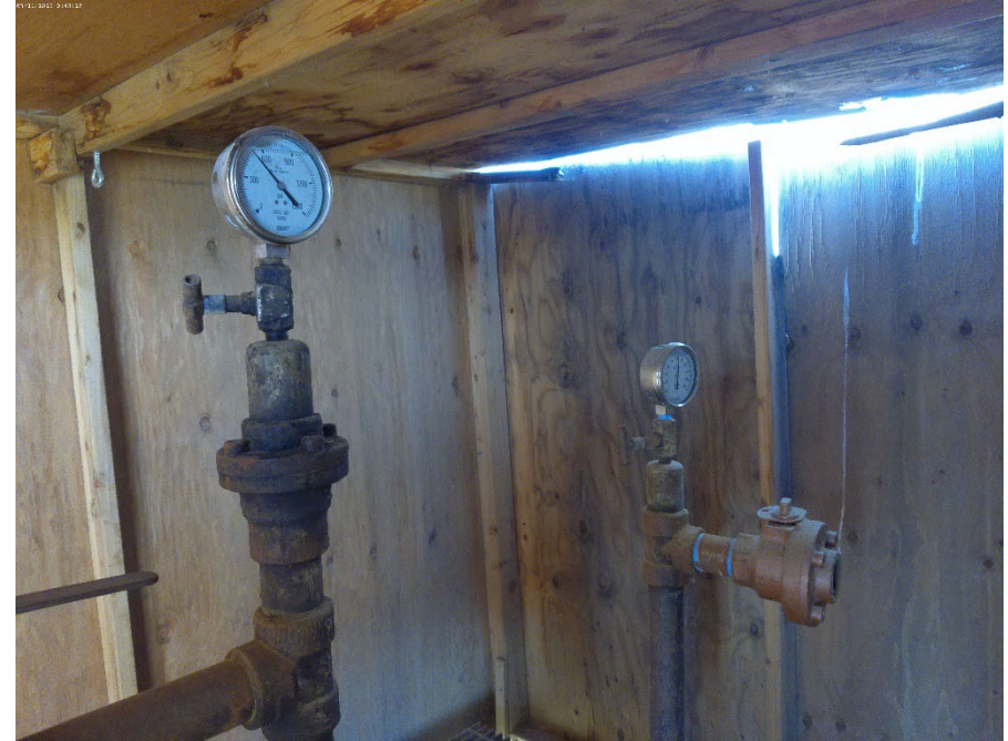
Injection Wellhead inside housing
