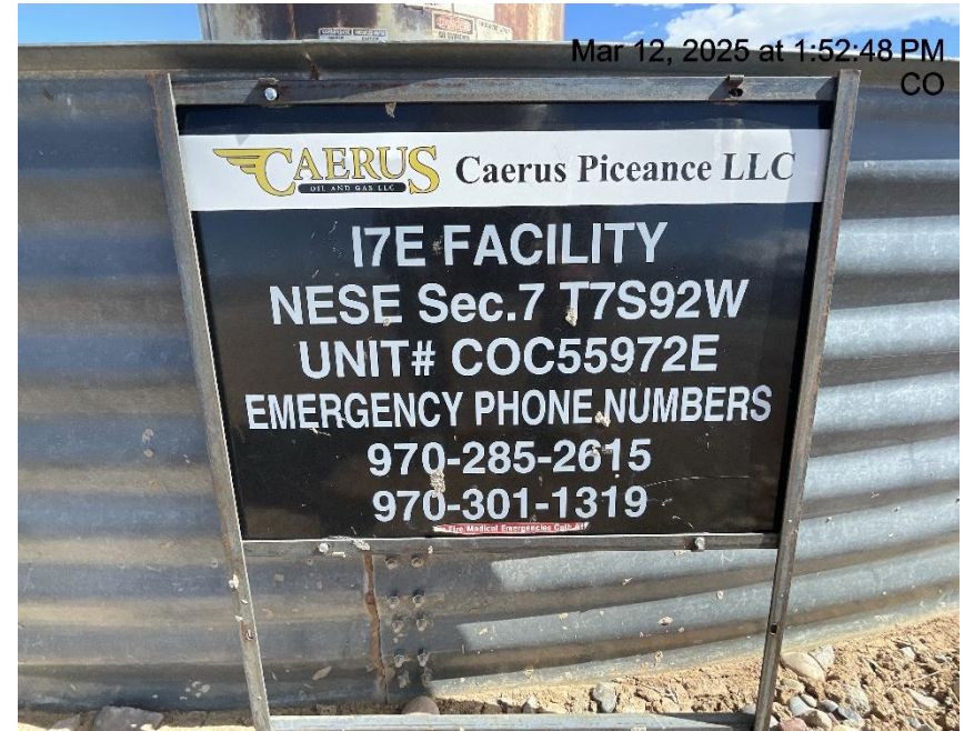
Photo # 2729 Battery sign missing required information/sign not in compliance with CECMC rules
