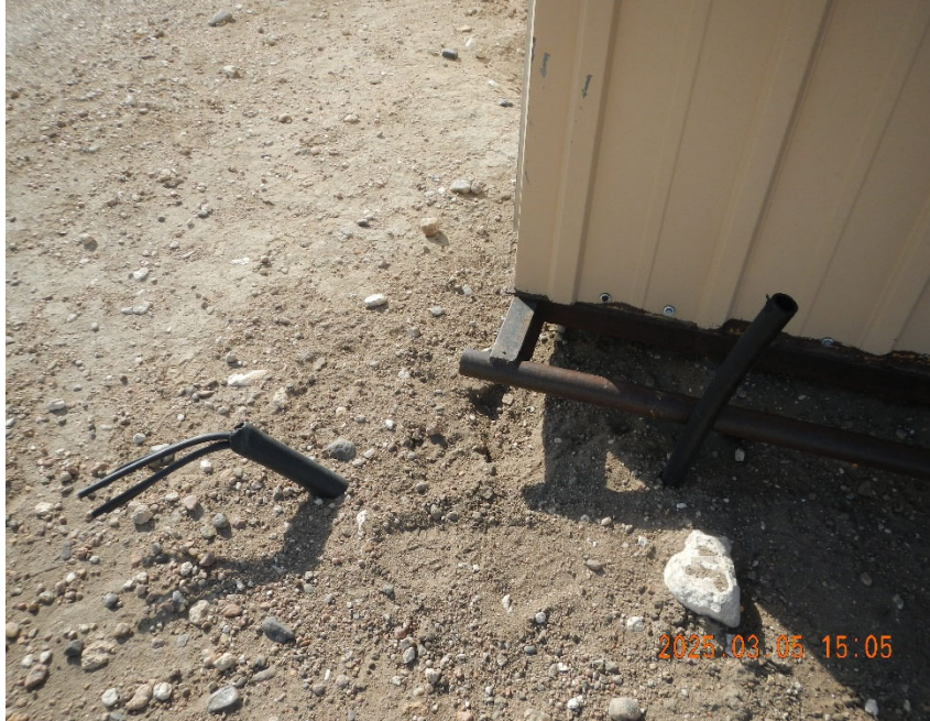
9. Stubbed up lines at meter shed.
