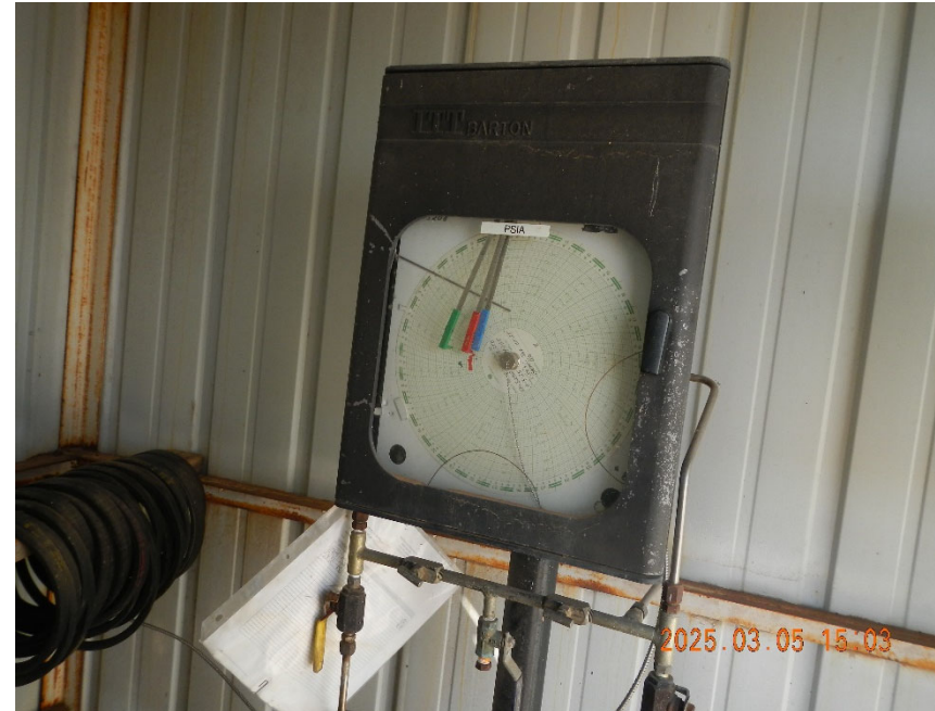
8. Gas meter inside meter shed.
