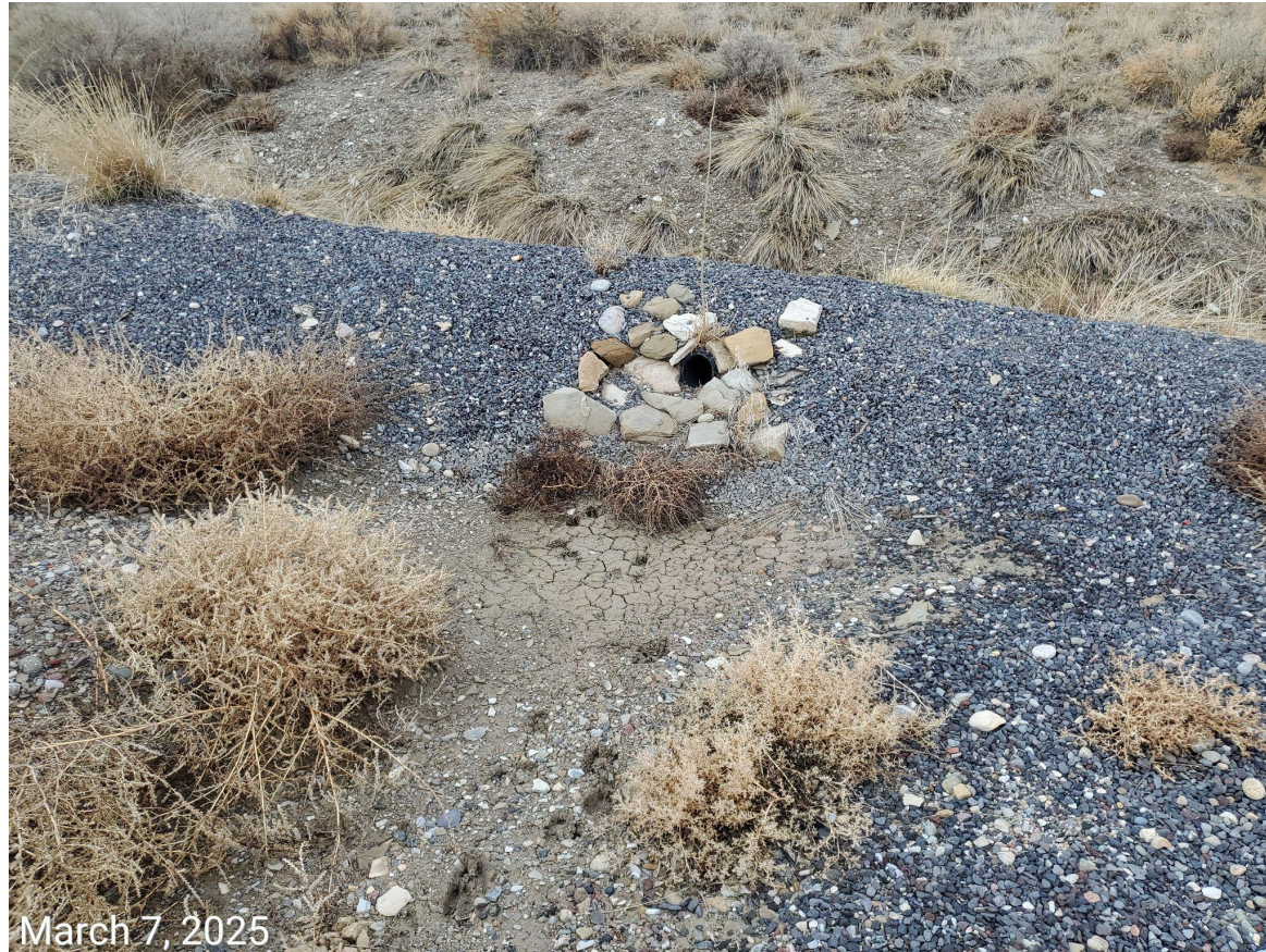
Photo 5: Photos shows sediment trap and outlet on the western working pad surface.
