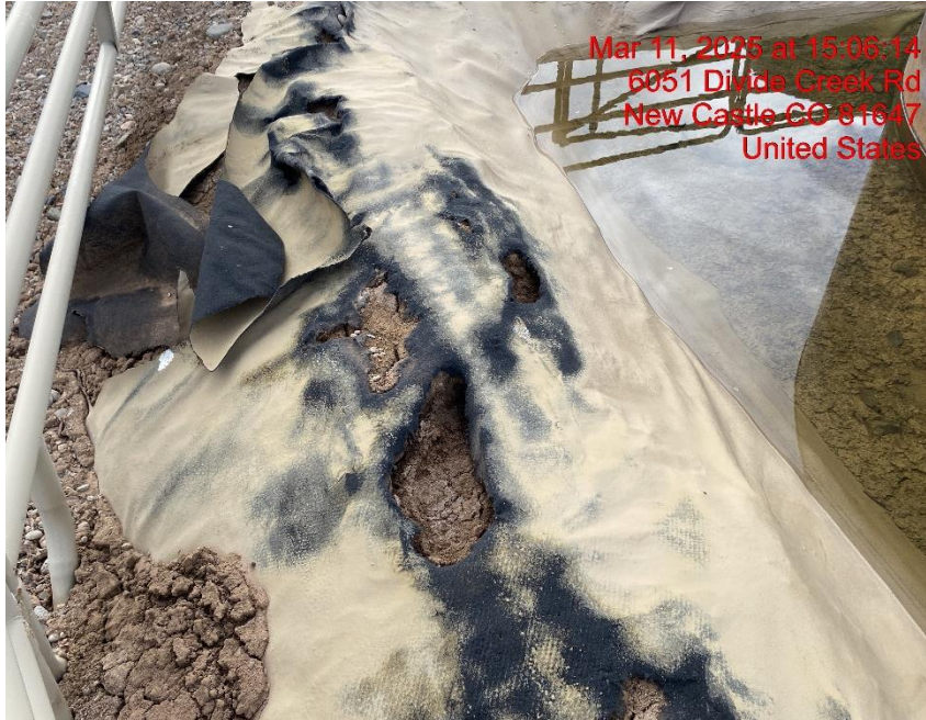
Unserviceable Berm Liner – Photo #07158
