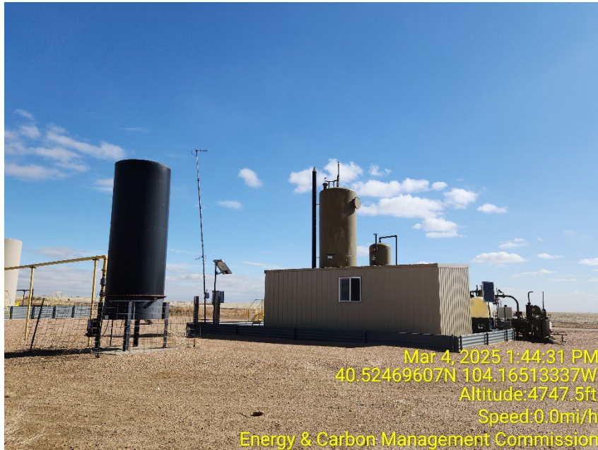
Photo 5 – Heater Treater and ECD
