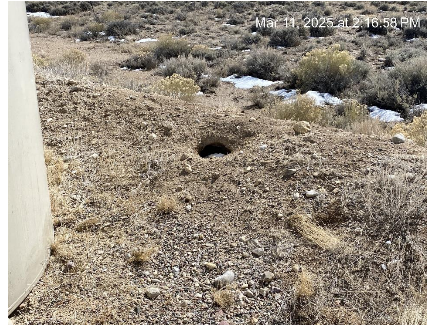
Berm capacity inadequate
